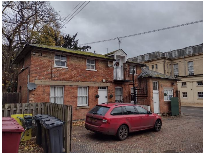
Figure 1: Southern elevation of building 1
