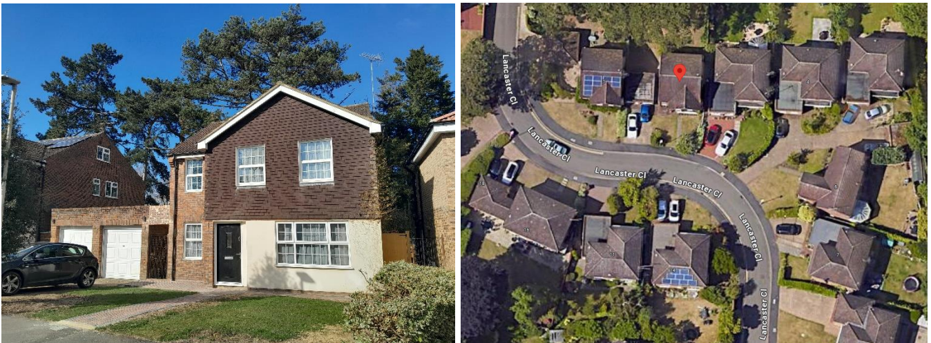
Fig 1 & 2: View from the front of the property (13/03/25); Image from Google Map (13/05/25)
