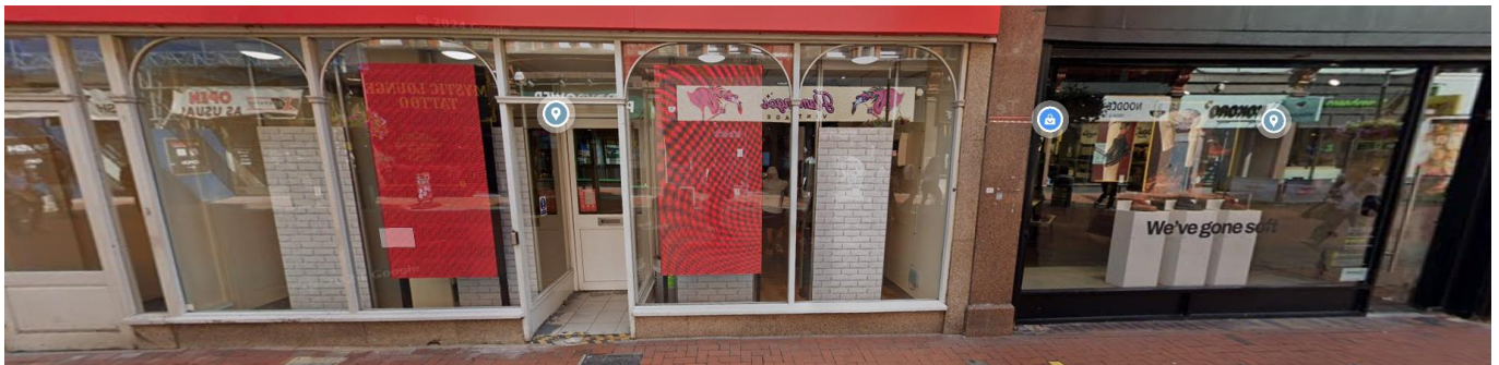
Figure 2 - Existing shop fronts to north of site
