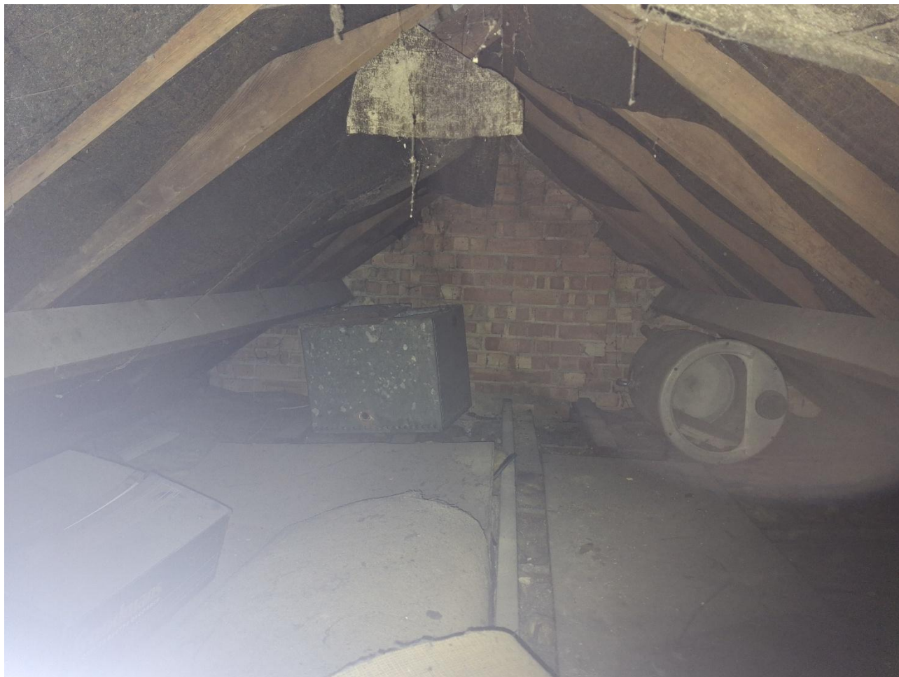
Figure 4: The loft void of B1
