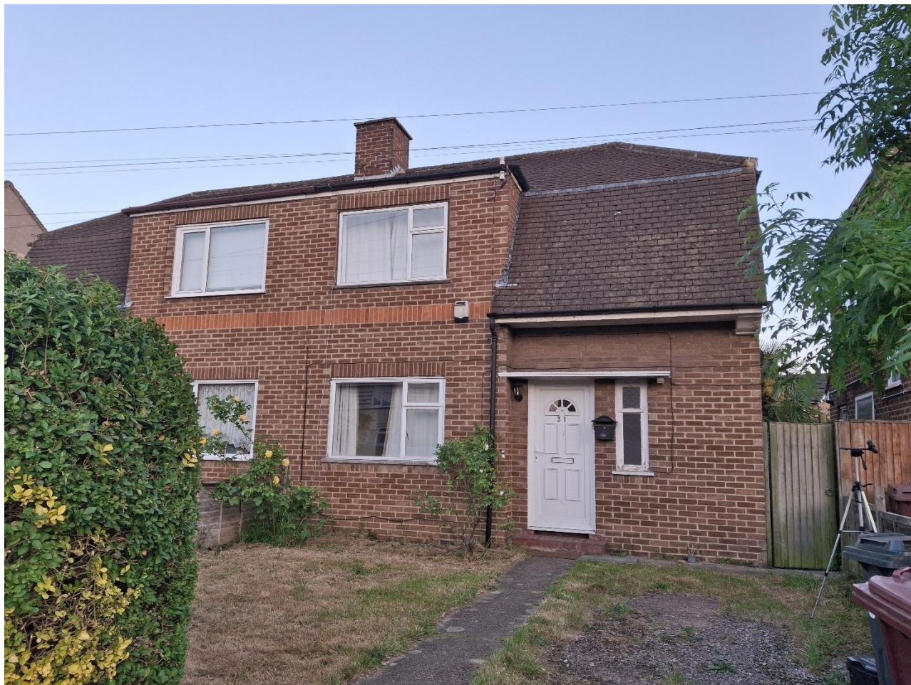
Figure 3: The front (north) of B1
