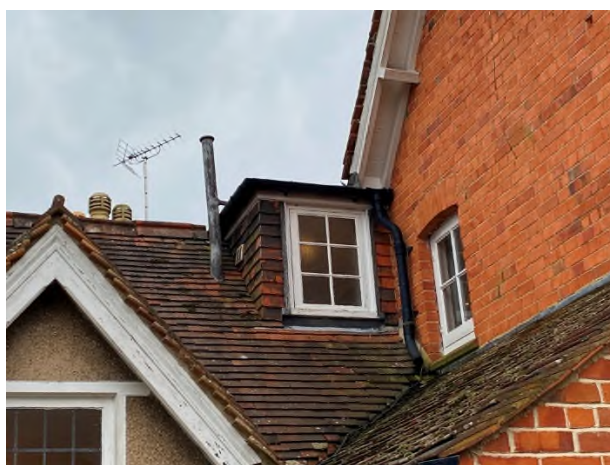
Figure 37: Dormer on the west side of the service wing roof
