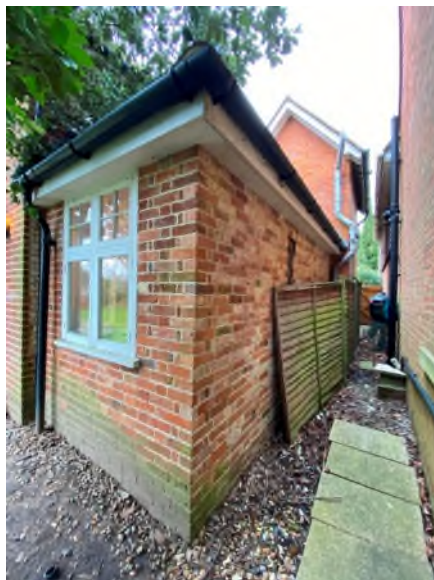
Figure 50: Brick extension replacing a conservatory on the east side of the east wing (2005)
