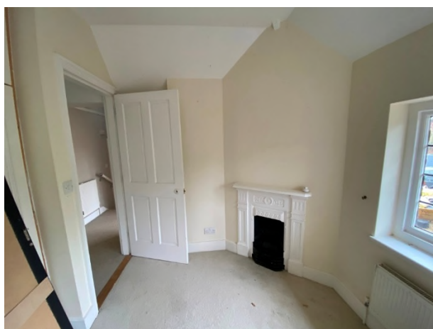
Figure 40: First floor of the 2-storey extension to the east wing
