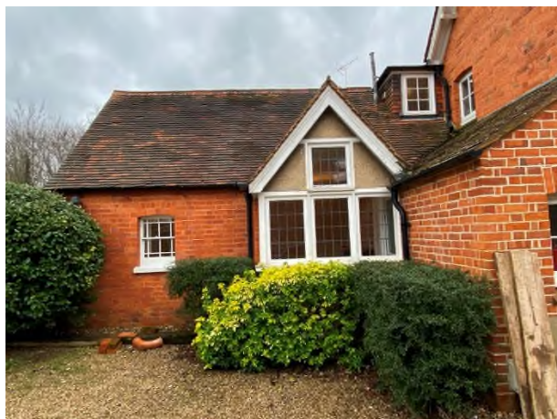
Figure 17: Single storey rear extension
