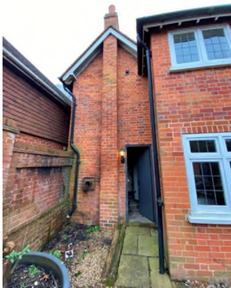
Figure 46: 2-storey side extension to the east wing
