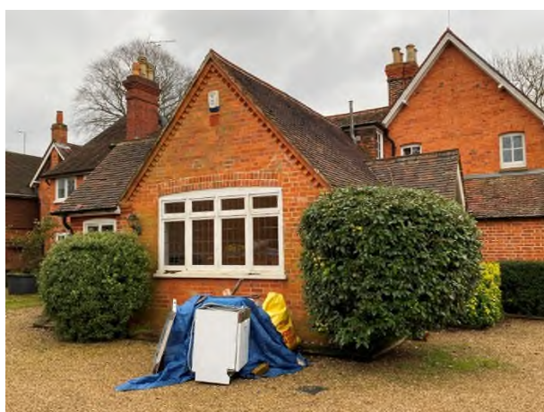
Figure 18: North elevation of the single storey rear extension
