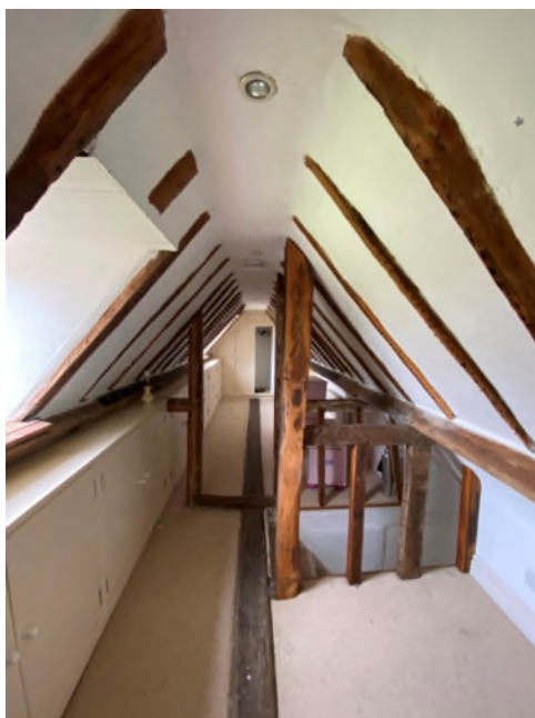
Figure 14: Attic of Phase 1
