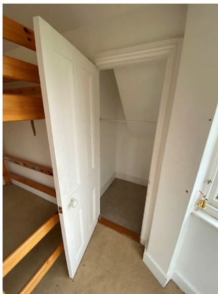
Figure 57: Door to a cupboard on the first floor of the central rear wing
