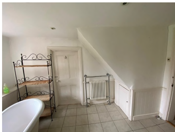
Figure 13: Eastern room on the first floor looking towards a 4-panel connecting door and later stair enclosure
