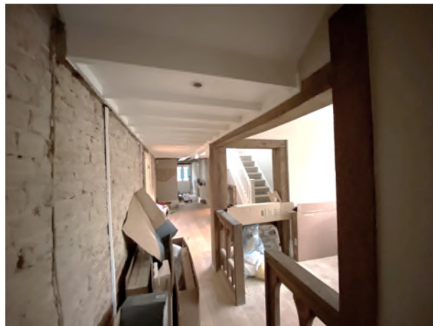
Figure 30: Phase 2 entrance hall
