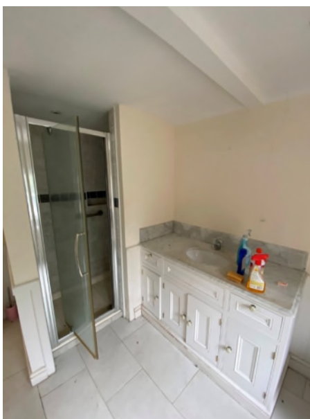
Figure 48: Bathroom on the first floor
