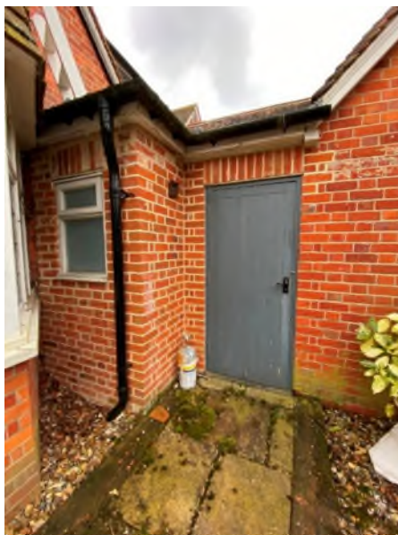
Figure 49: Modern infill of the area between the service wing extension and the staircase extension
