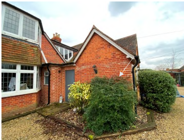
Figure 45: East elevation of the extension to the service wing
