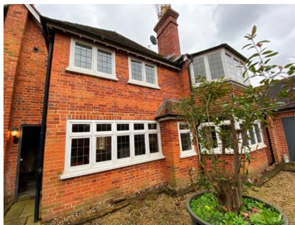
Figure 35: 2-storey rear extension
