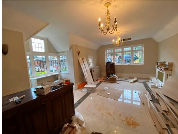
Figure 29: Ground floor of the single storey rear extension looking north
