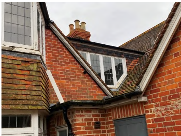
Figure 36: Extension housing the existing staircase
