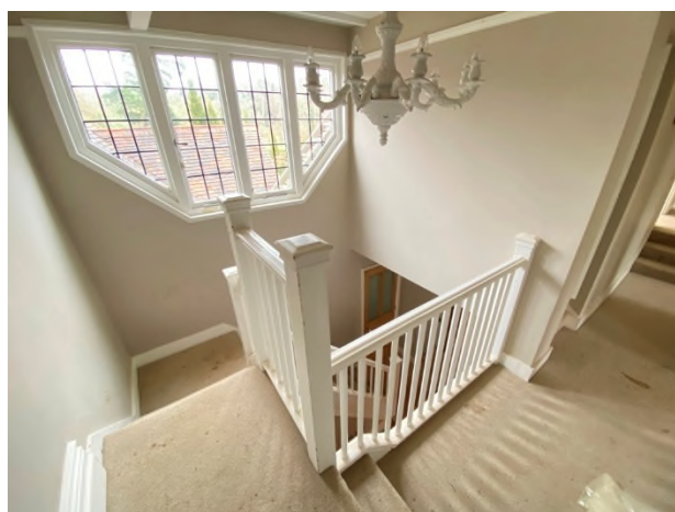
Figure 44: Staircase viewed from the landing
