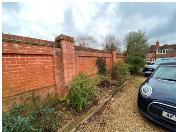
Figure 51: Modern brick boundary wall
