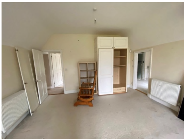
Figure 23: View towards a removed staircase and internal partition wall looking north on the first floor of the east wing
