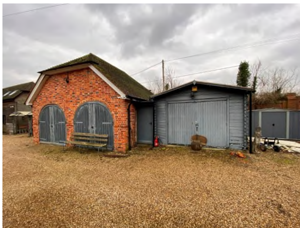
Figure 52: Modern garage to the north-west of the house
