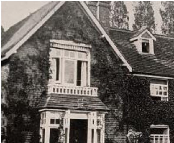
Figure 9 - Photo showing former balustrade over bays
