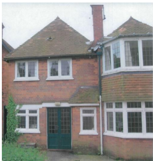
Figure 7 - Former French double doors on North Elevation
