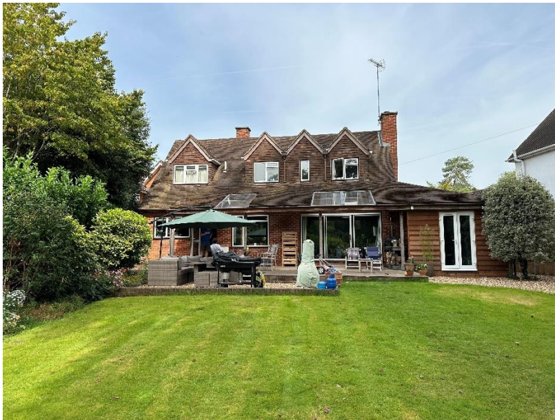
Figure 4 - South elevation of Kingfishers Reach
