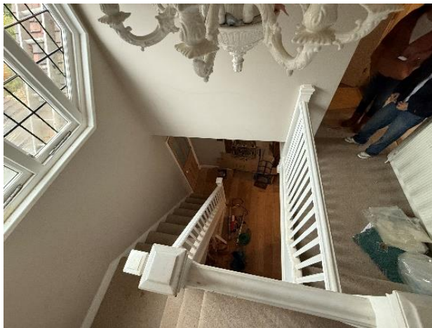
Figure 10 - Existing Staircase - View 1
