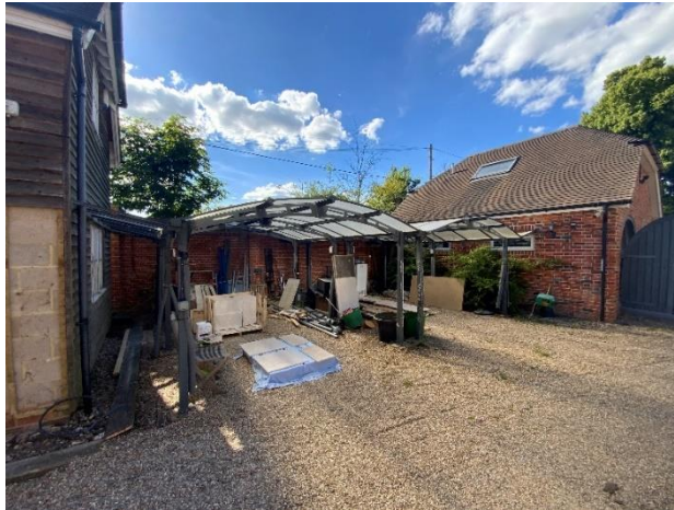
Figure 13 - Carports to be demolished
