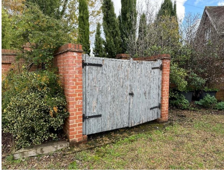
Figure 12 - The oil tank compound to be removed
