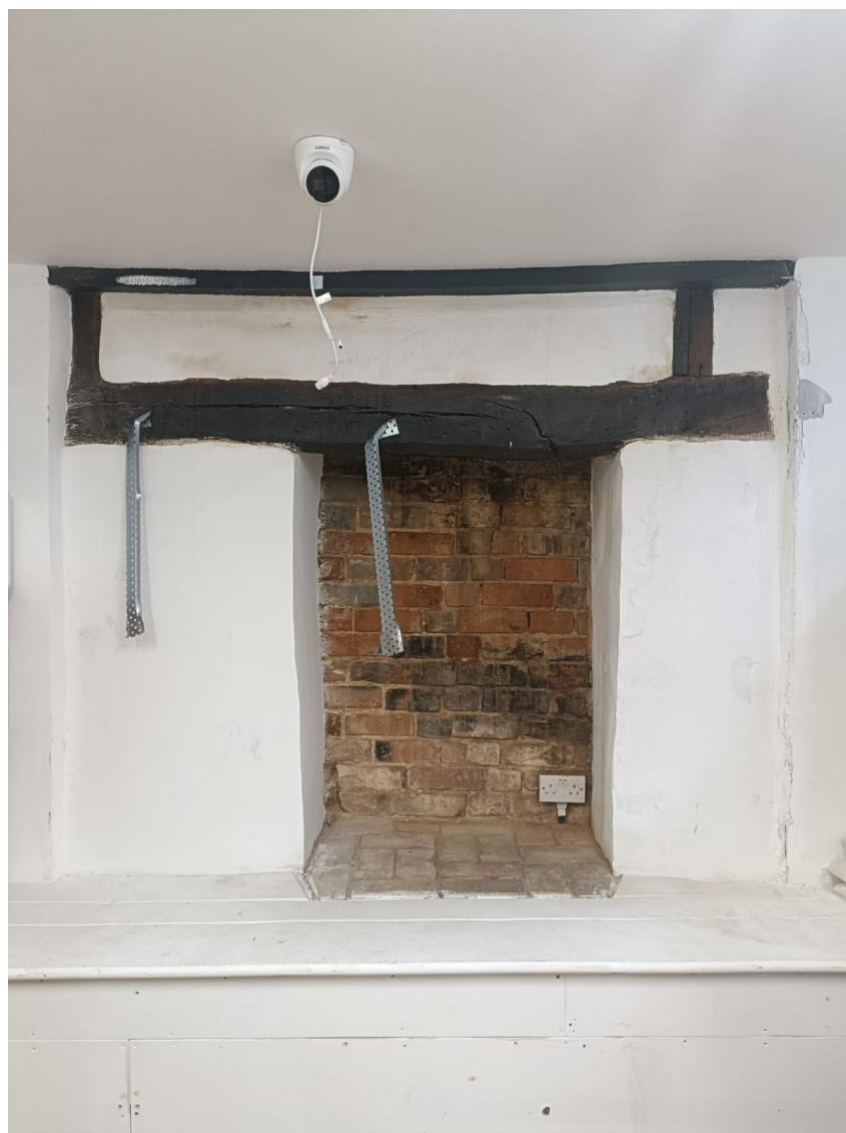
Picture 1, Open fireplace at the rear of number 35's rear wing wall
