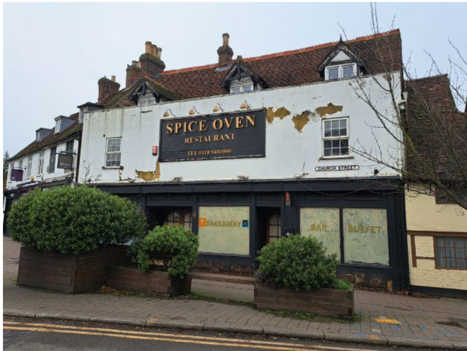
Photo 1 – View of front (south) elevation
