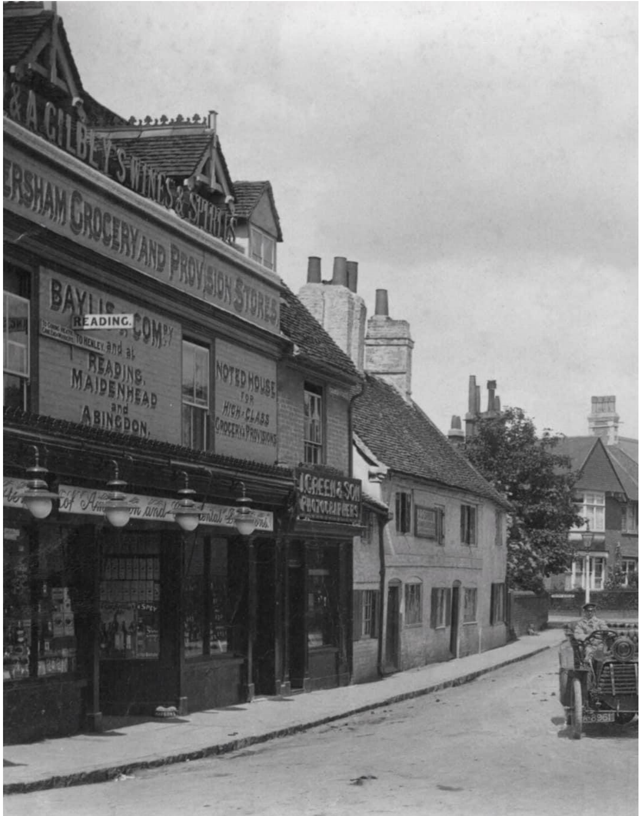
Photograph of the property in approximately 1901- Note the width of the parapet detail, the middle sash window and the shop detailing.
