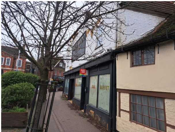
Photo 8 – View of front/side elevation (southeast)
