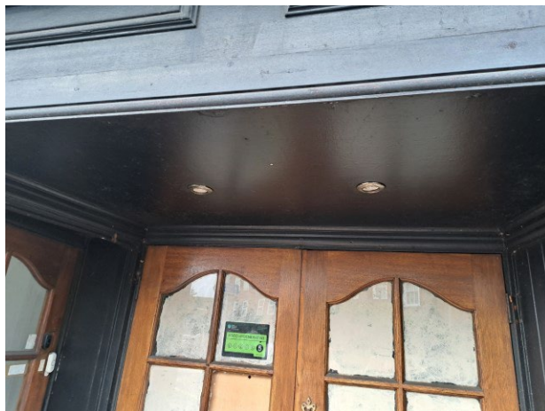
Photo 3-5 – View of main entrance way
