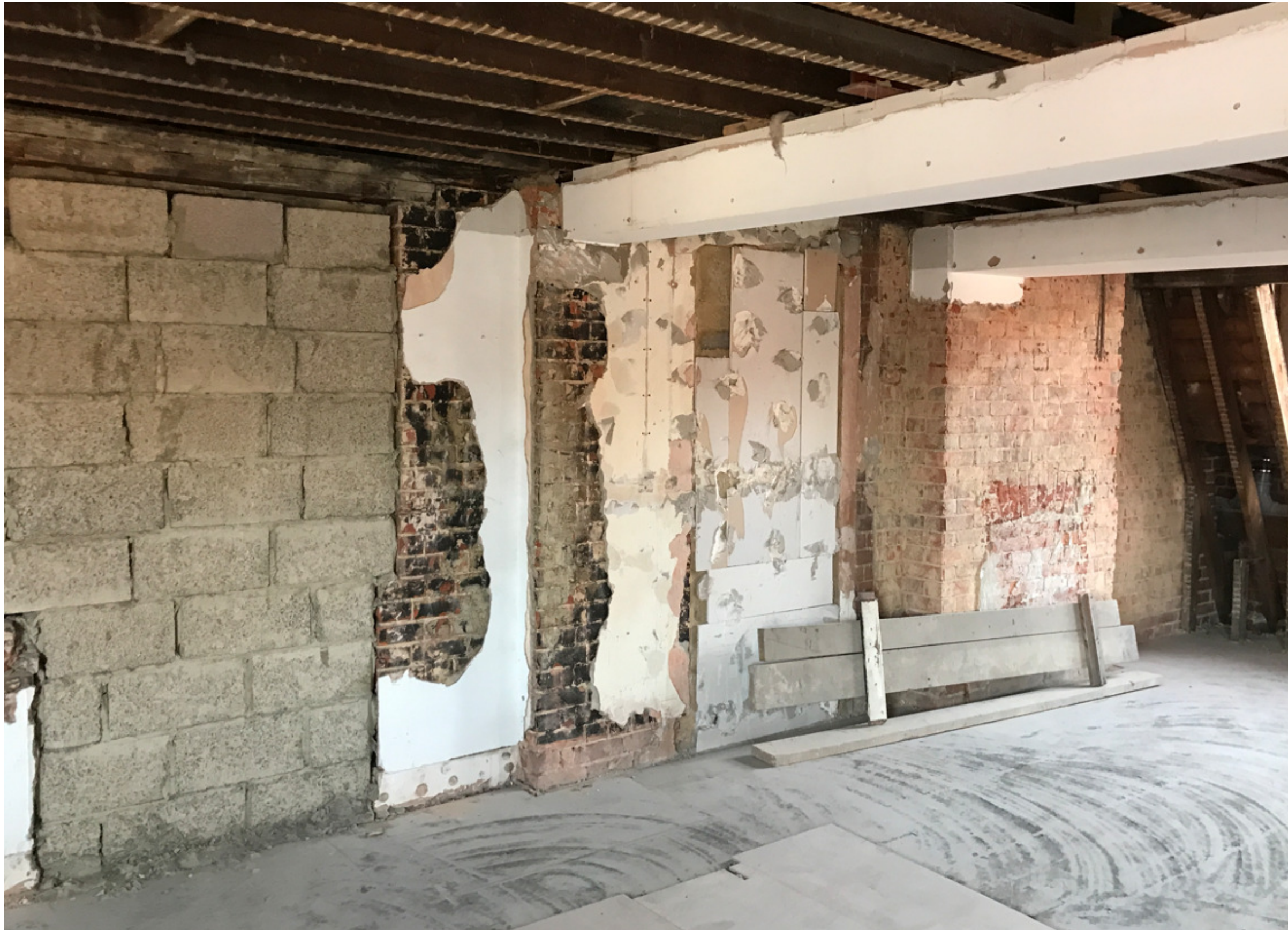
Existing Typical Internal Party Wall :
