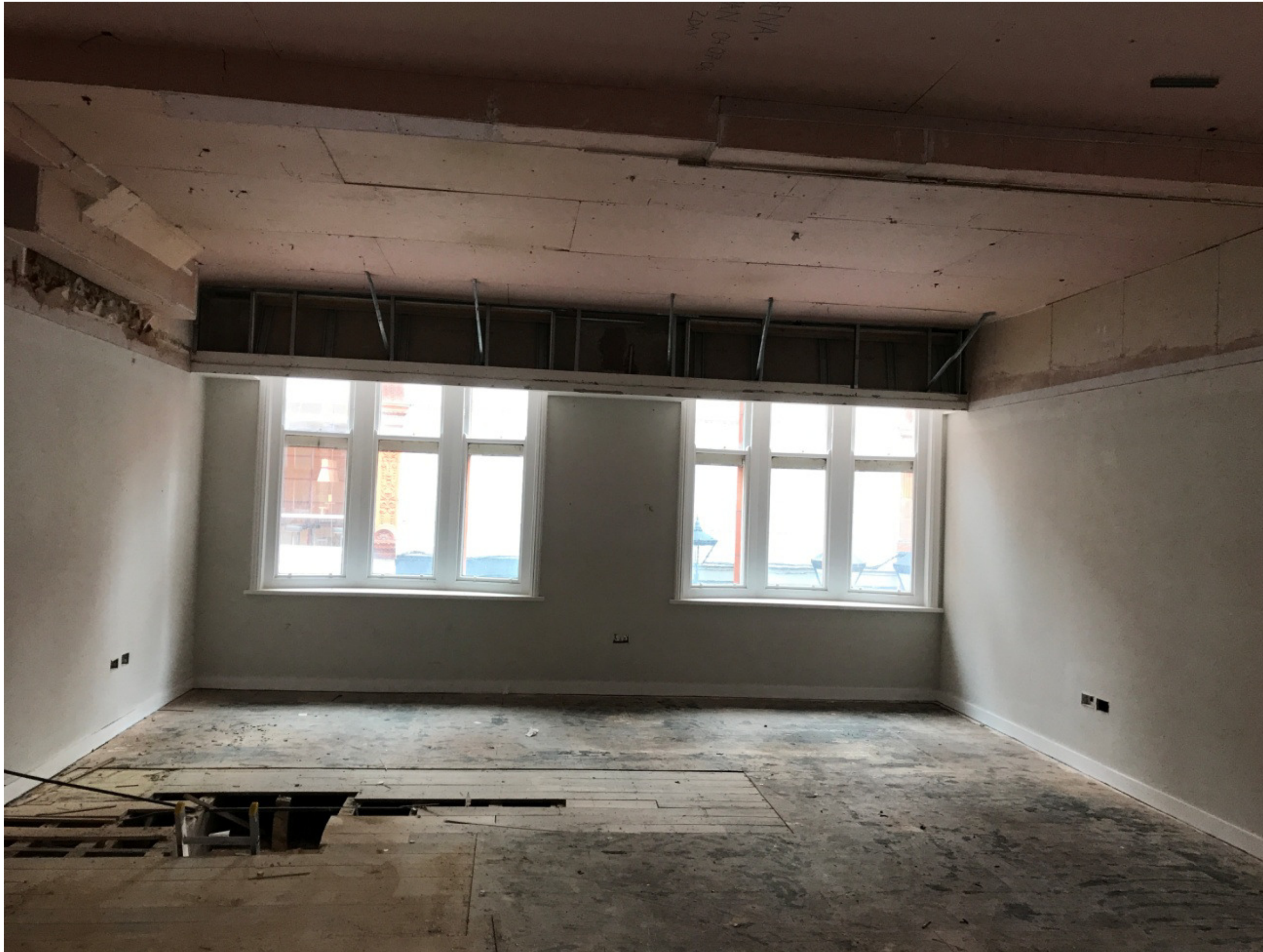
Typical existing first, Second & Third Floors – Looking towards Queen Victoria Street:
