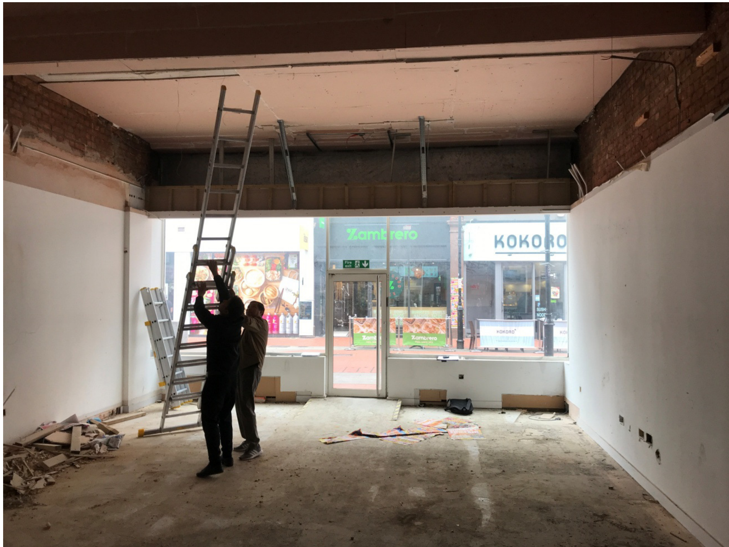
Existing Ground Floor Level – Existing Retail Unit – Looking towards Queen Victoria Street:
