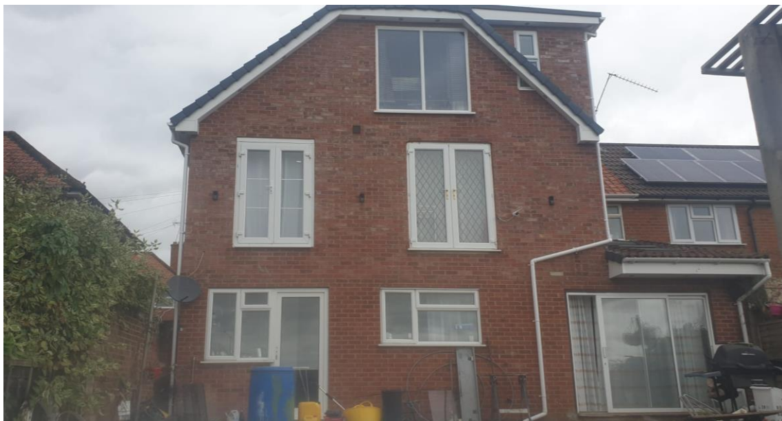
Rear Elevation of No. 10 Anglefield Road
