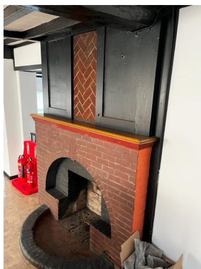
Figures 14 and 15: 20 th century chimney piece applied to the 17 th century stack (ground floor) and 17 th century winder stair between the first and second floor
