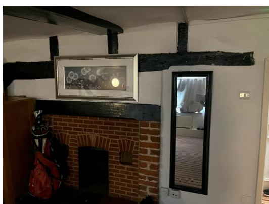
Figures 16 and 17: Exposed timber framing present within the main first floor room
