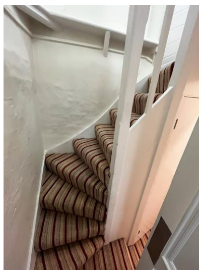
Figures 14 and 15: 20 th century chimney piece applied to the 17 th century stack (ground floor) and 17 th century winder stair between the first and second floor
