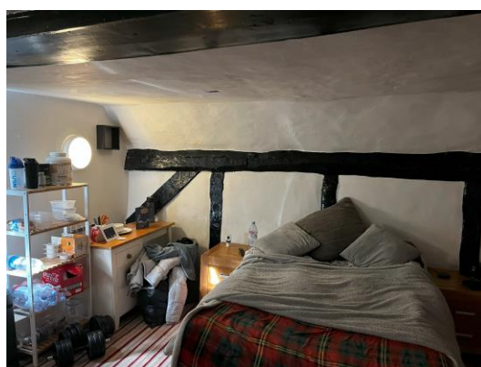
Figures 16 and 17: Exposed timber framing present within the main first floor room
