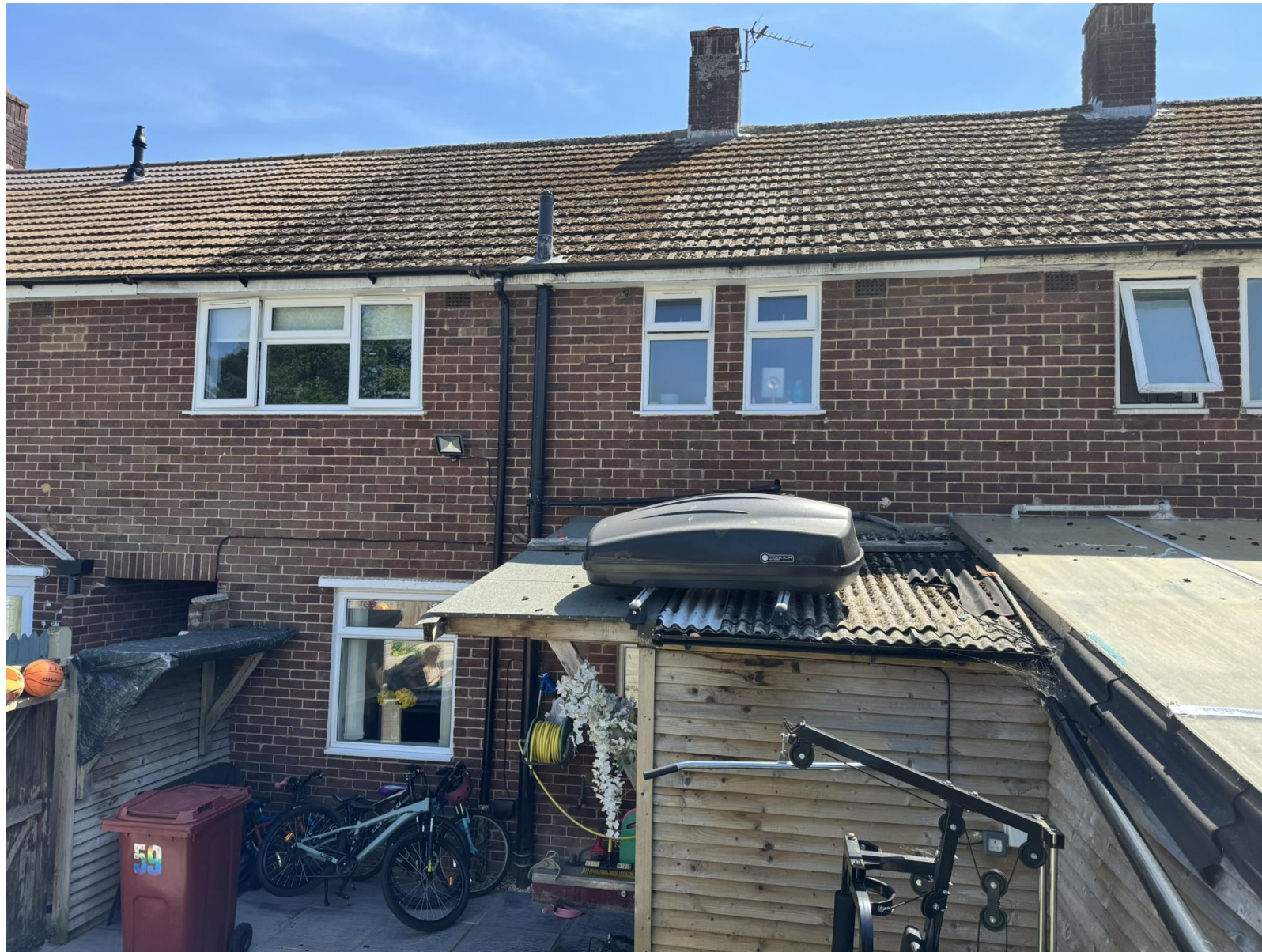
Site Visit Photos – taken on the 14 th of May 2025
