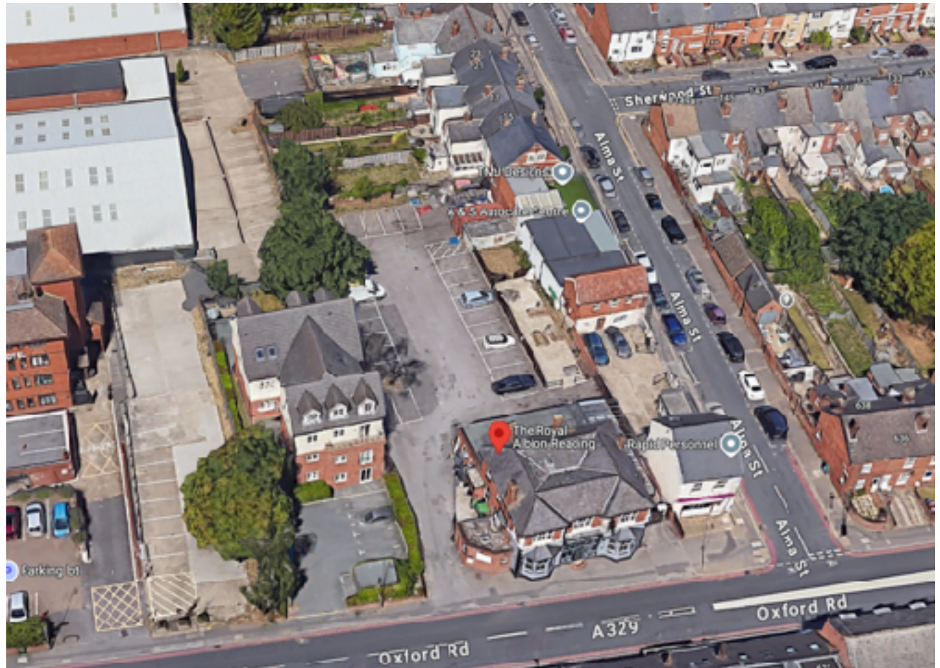
Fig 1: Aerial view of site
