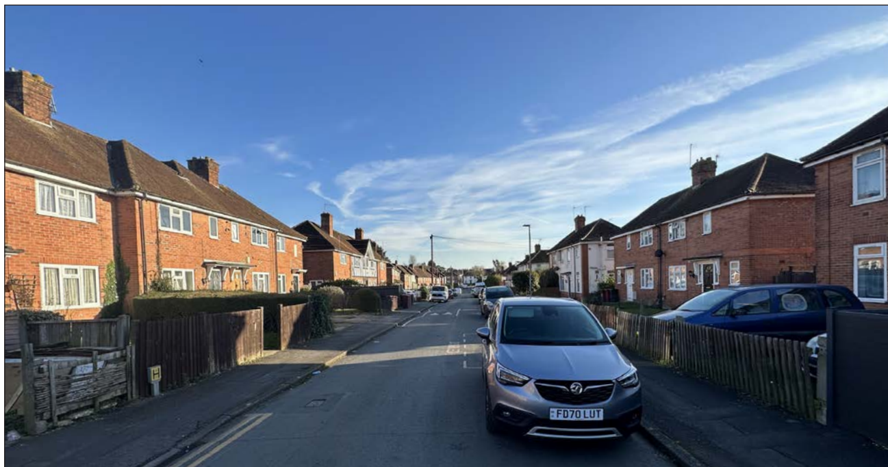
FIGURE 05 View of the earlier side extension from the front of the property facing east
