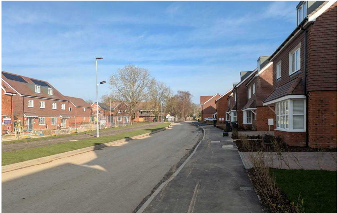
Photo 4.2 - The Fairway, looking east
