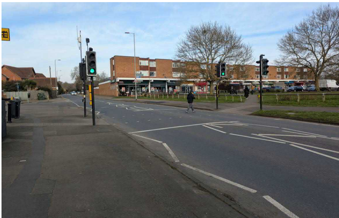
Photo 4.7 - Peppard Road signalised crossing, looking north towards the local centre
