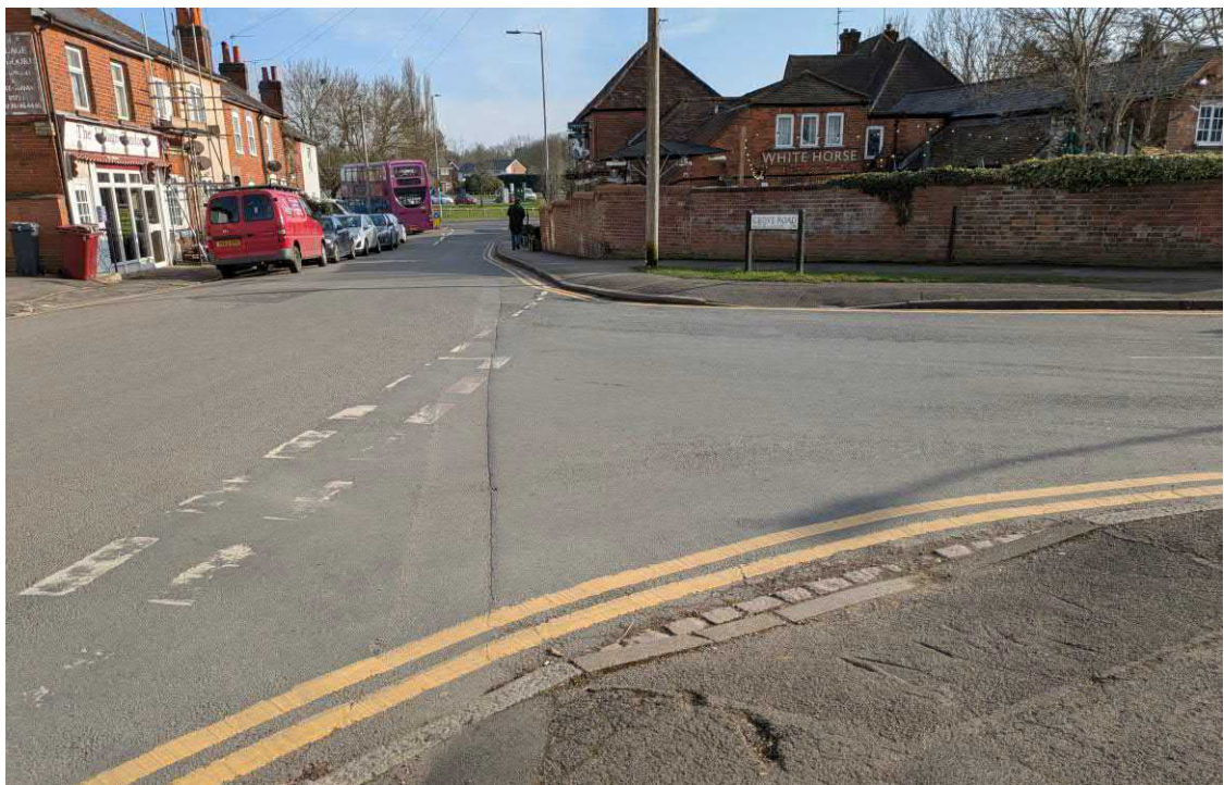
Photo 4.3 - Junction of Kidmore End Road and Grove Road, looking south
