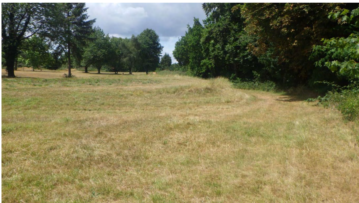
Plate 7.15: Land levelling in north-west of the Site
