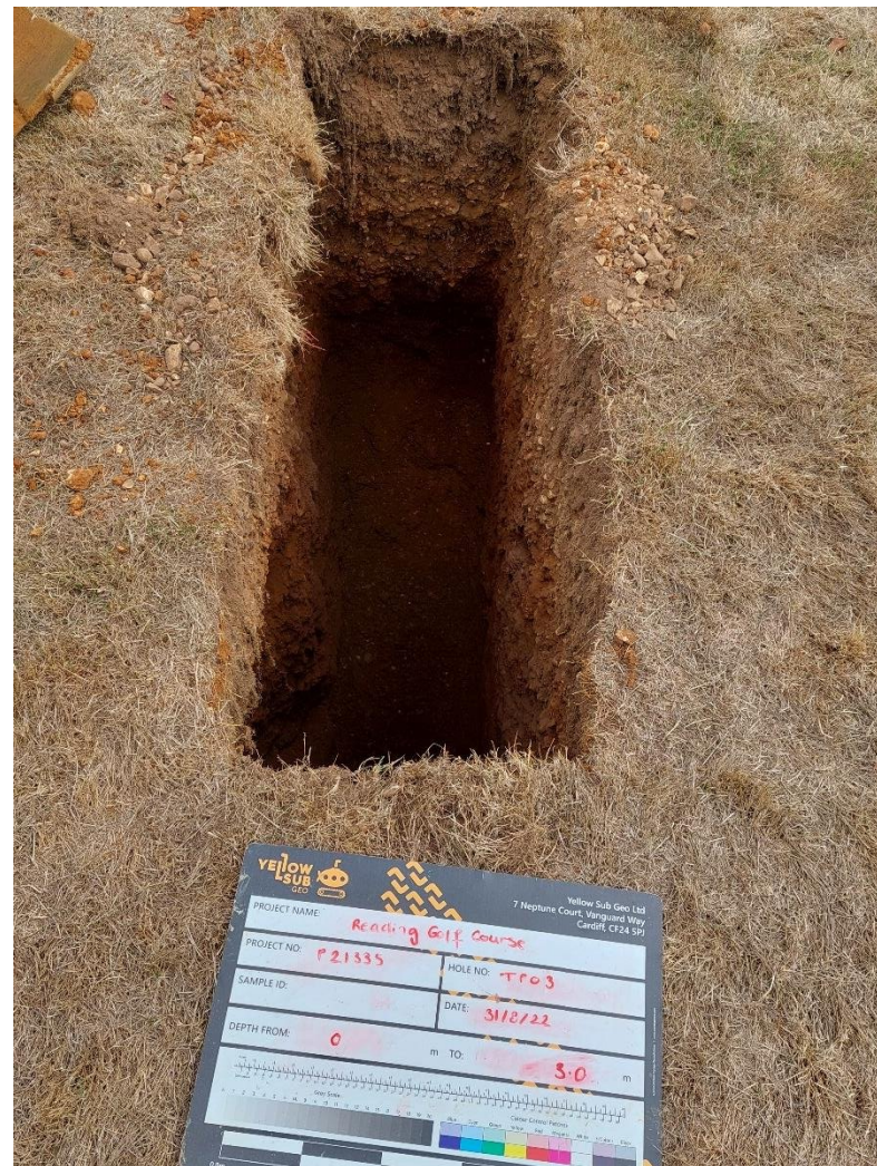
TP03 trial pit
