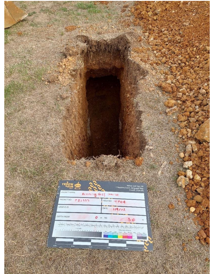
TP04 trial pit
