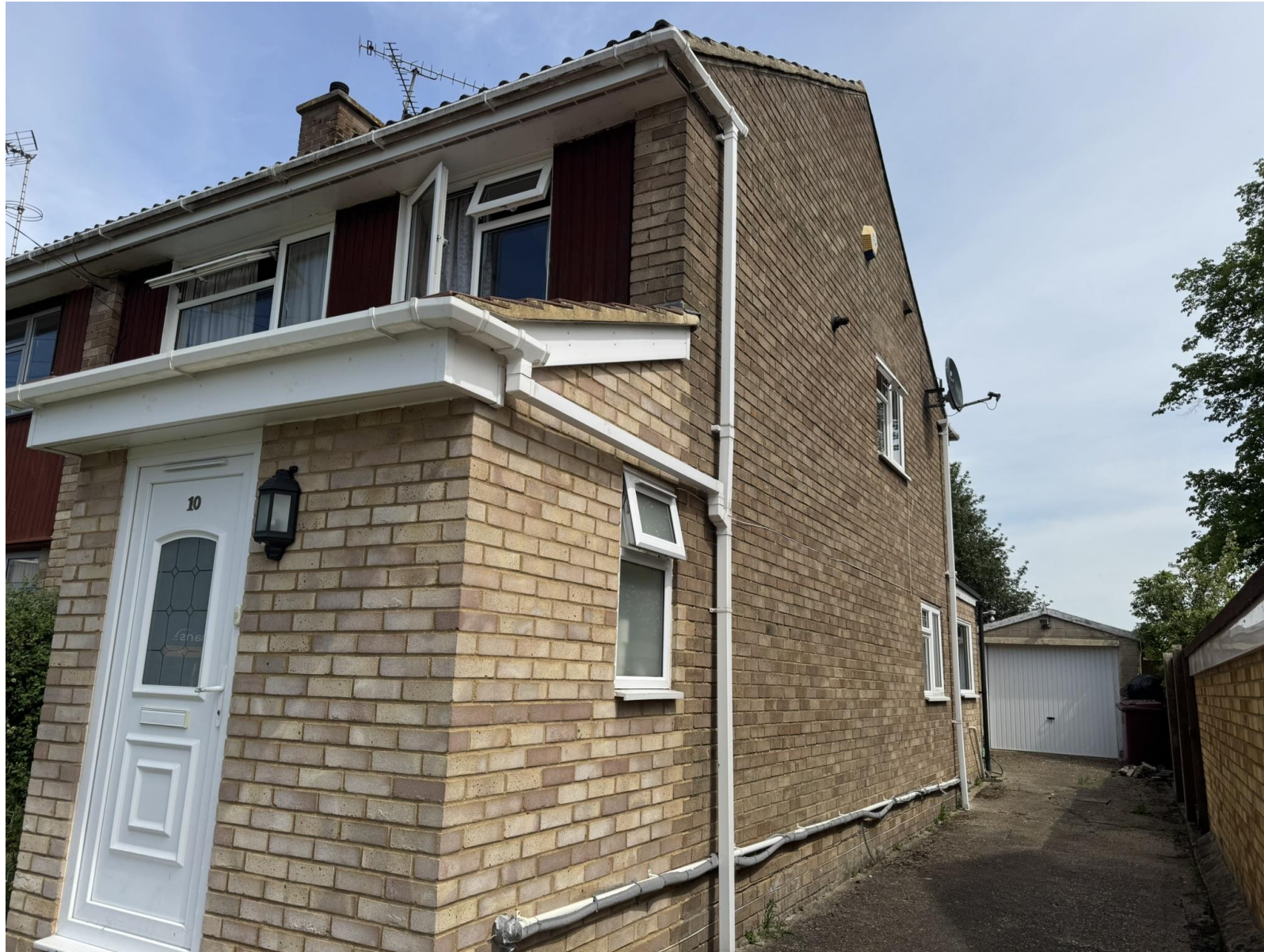
Site Visit Photos taken on 1 st of May 2025
