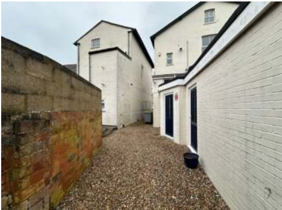
Photograph 10: Yard area situated between the existing structures, facing south.
