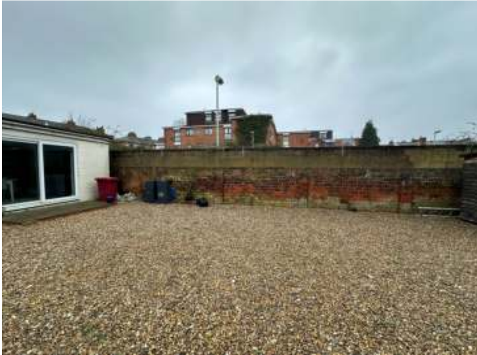
Photograph 9: External area directly to the rear of no. 134, including the single story extension of the building, facing west.
