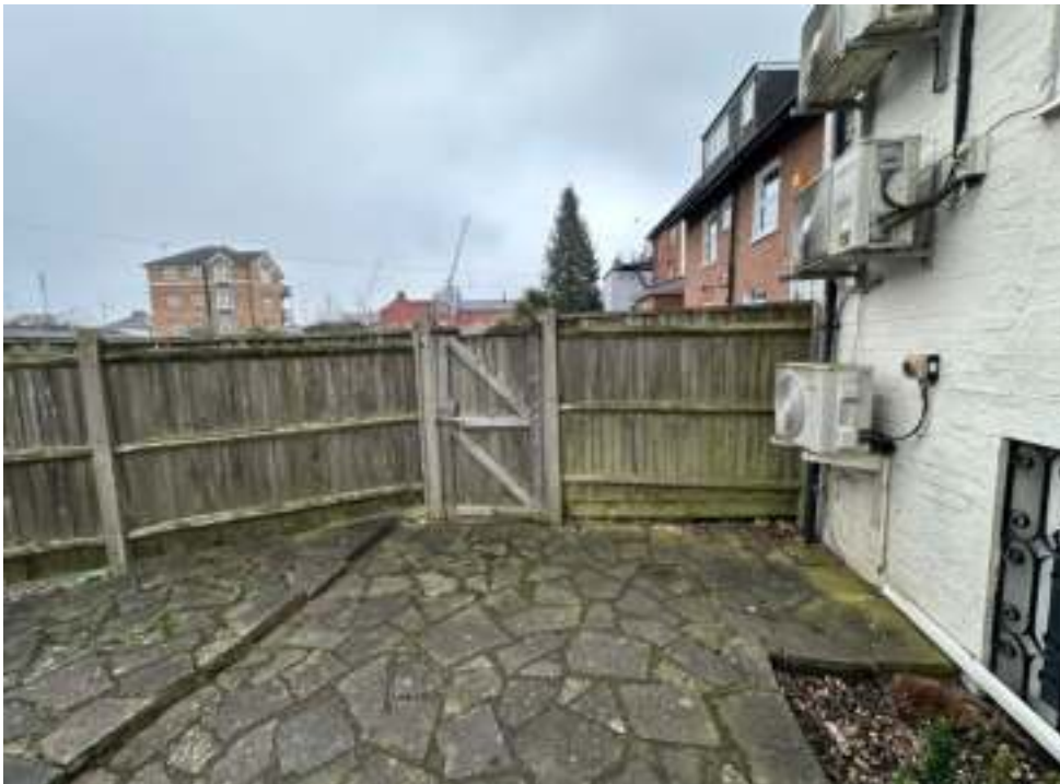
Photograph 6: Rear of no. 132, including hardstanding yard area and neighbouring residential land use (facing east).
