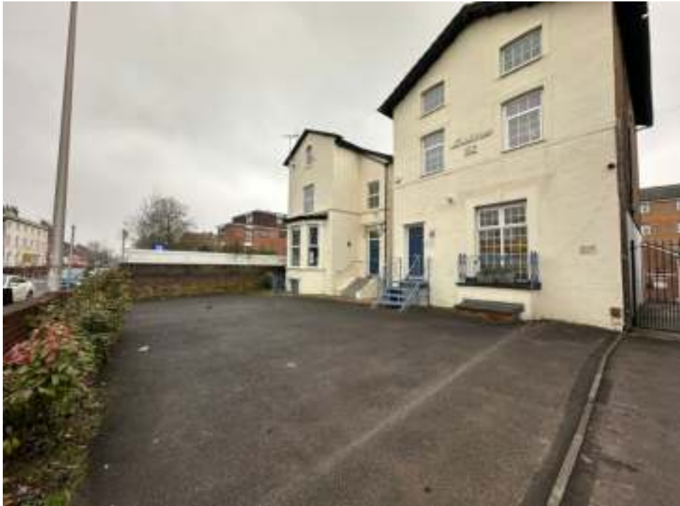
Photograph 3: Front facades of the existing buildings in the south of the site, facing northwest.
