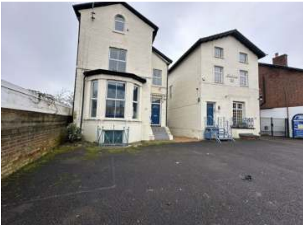
Photograph 2: Front facades of the existing buildings in the south of the site as seen from Oxford Road, facing north/northeast.
