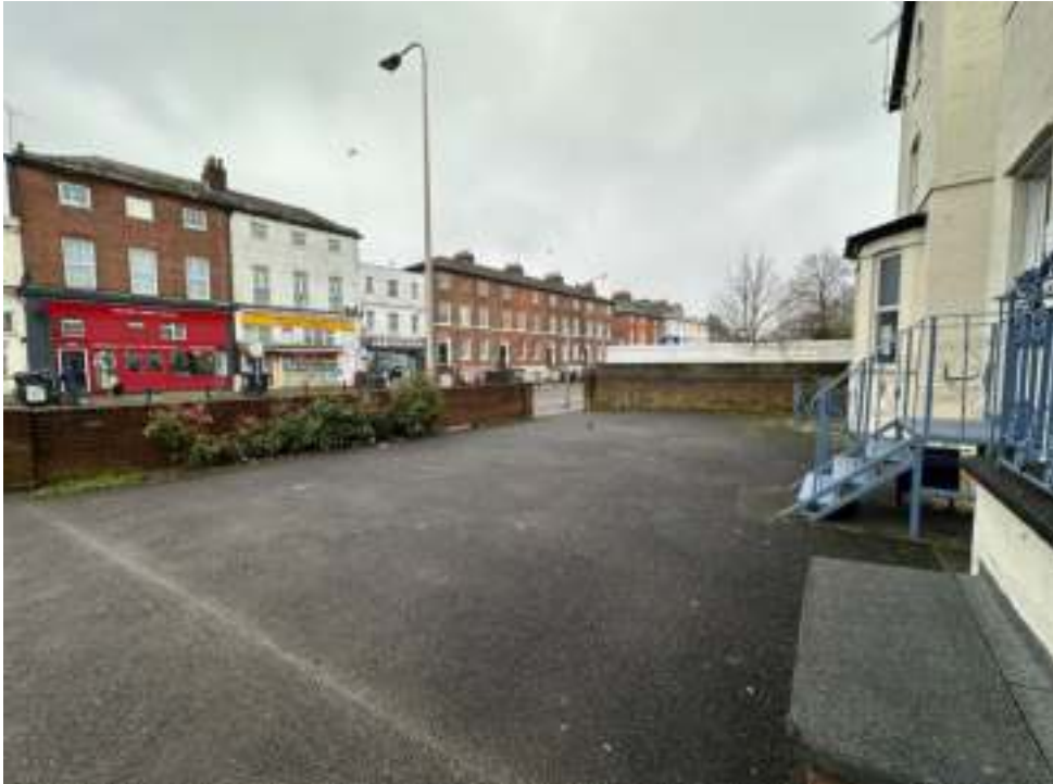
Photograph 1: Hardstanding / car parking area to the front of the exiting buildings in the south of the Site as well as neighbouring residential and commercial land use (facing southwest).
