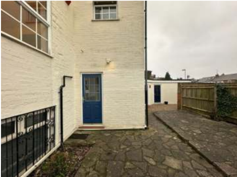
Photograph 5: Rear of no. 132, including hardstanding yard area (facing west).
