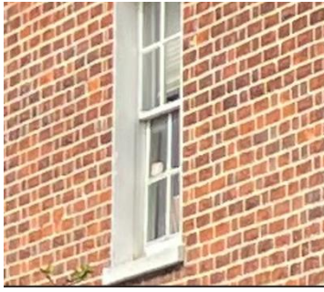
To show the south elevation of the listed building at 101 Oxford Road
