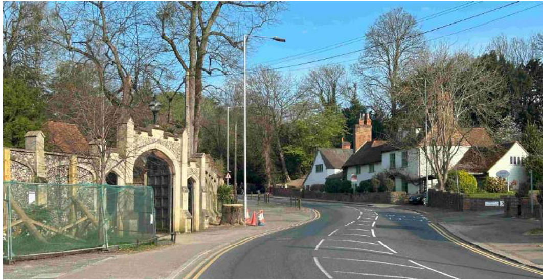
Caversham Court eastern boundary wall along Church Road with Banksfoot, a Grade II listed early to mid C18 dwelling
