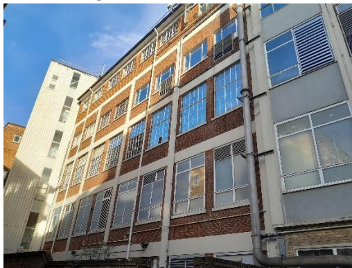
Fig 1. View from the west of 41 Minster Street. Site photo taken on 19/12/2024.
