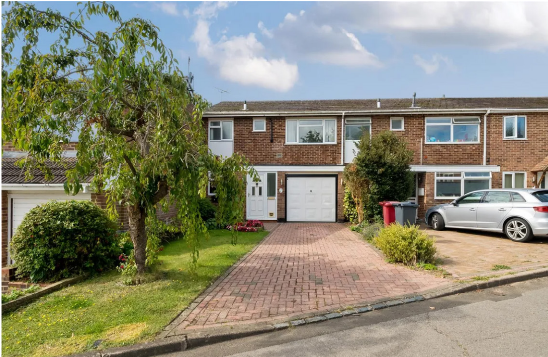
03 Front Driveway, Garden and Facade
