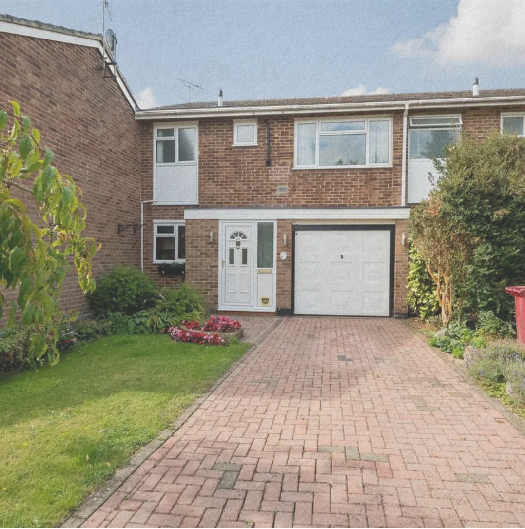
Existing Front Facade
