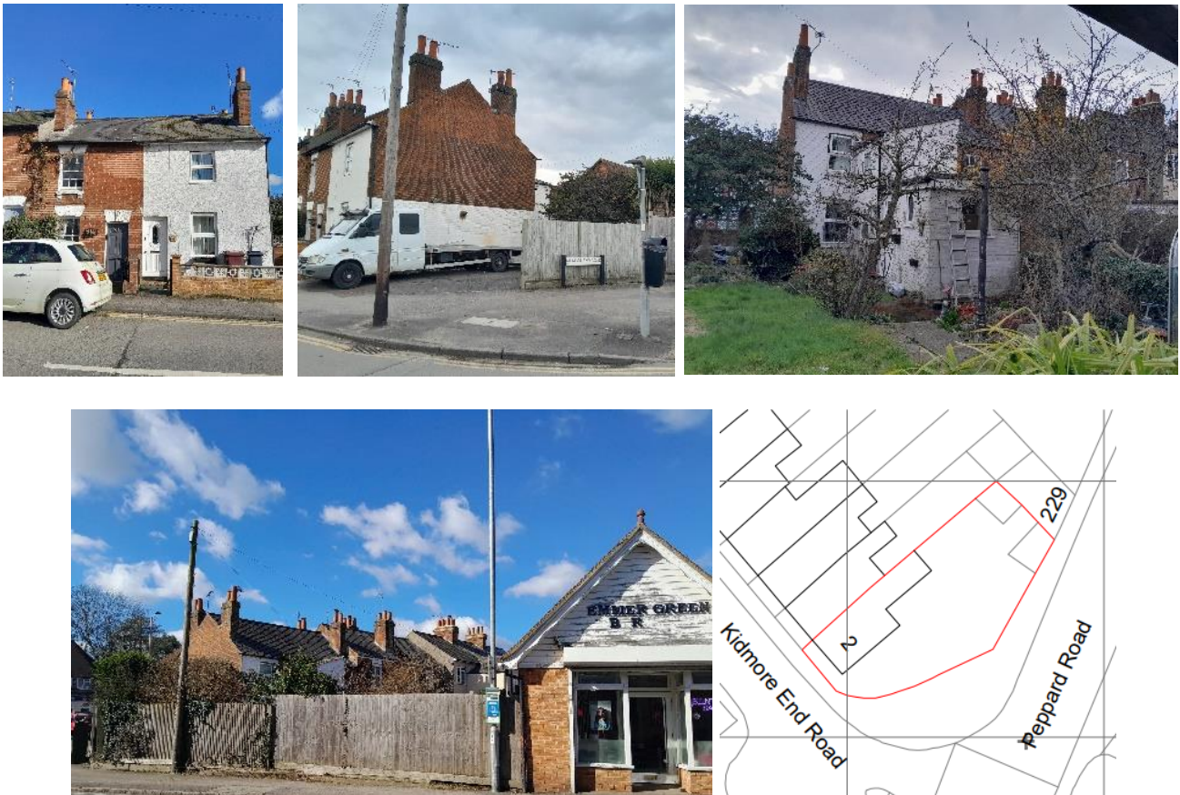
Fig 1-5: Views from front, side and rear of the property, taken on 27/02/25, and site location plan
