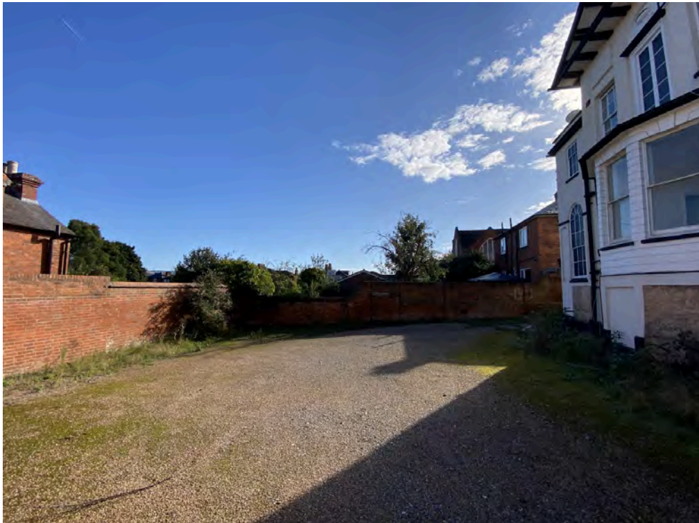
Photographic plate showing the rear of 2 Tilehurst Road (ROAVR, 2024)
