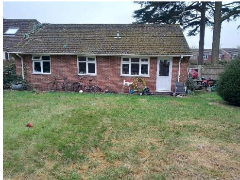
Looking towards rear elevation of existing bungalow
