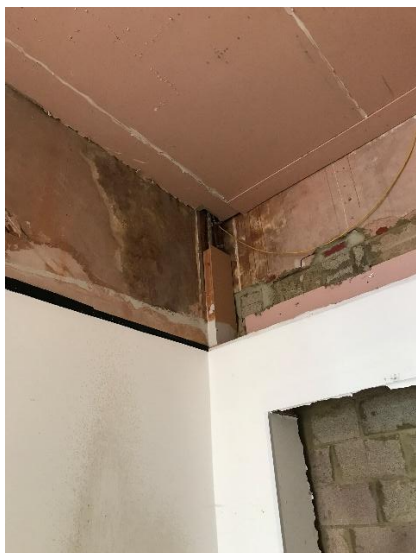
Plate 6. A detail of the modern finishes (plasterboard, blockwork and gypsum).
