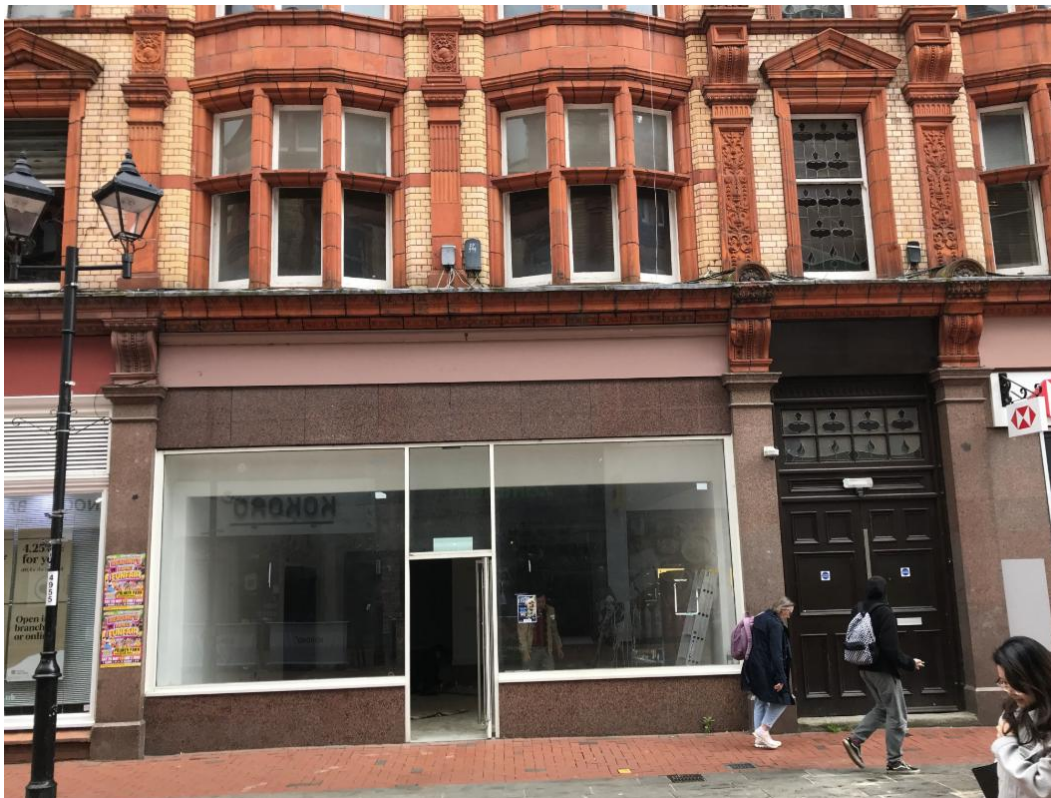
Plate 2. The existing shopfront, of poor quality relative to the age and architectural language used for the building above, illustrating a relatively modern insertion with fascia, sub-fascia and pilasters. The stallriser is evident (in contrast to that adjacent) although clad in modern materials. The historic entrance to the upper floors is evident to the right of the image.
