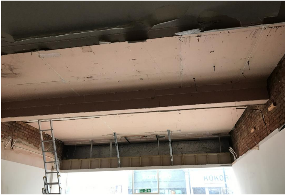
Plate 8. Plasterboard ceilings and encased beams. Any decorative cornices or other plasterwork is no longer present. The image shows the line of the previously suspended ceiling.
