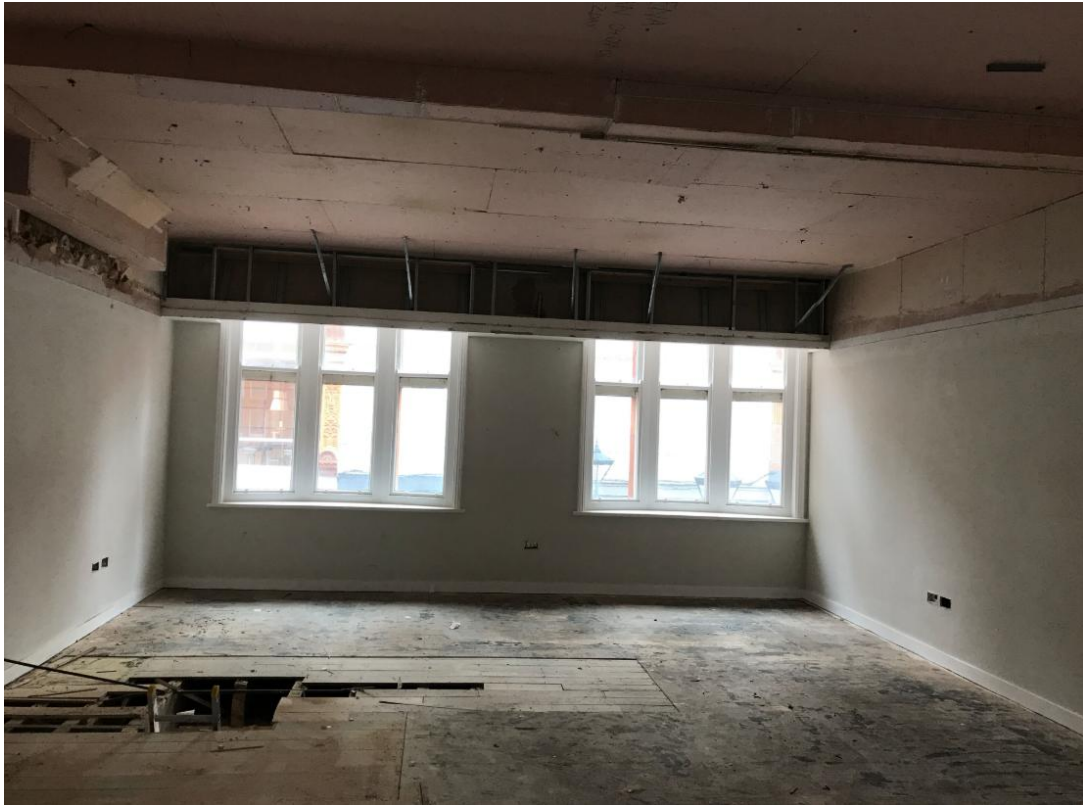
Plate 10. The first-floor front windows and evidence of over boarding of the 19 th Century floor boards. The ceilings however reflect those of the ground floor.
