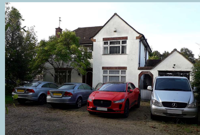
Figure 5: 47 Parkside Road (© Google St View)
