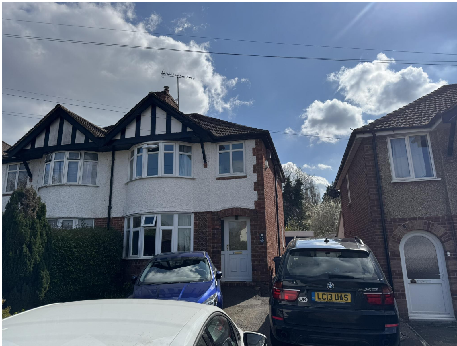
Site Visit Photos taken on 26 March 2025 by the assigned Planning Officer
