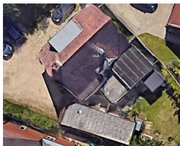
Google Earth aerial image
