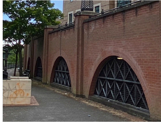
Railing precedent: existing railings and metal screens to the basement and riverside of the site
