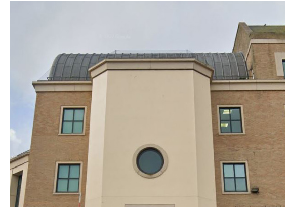
View of the East terrace from Gas Works Road
