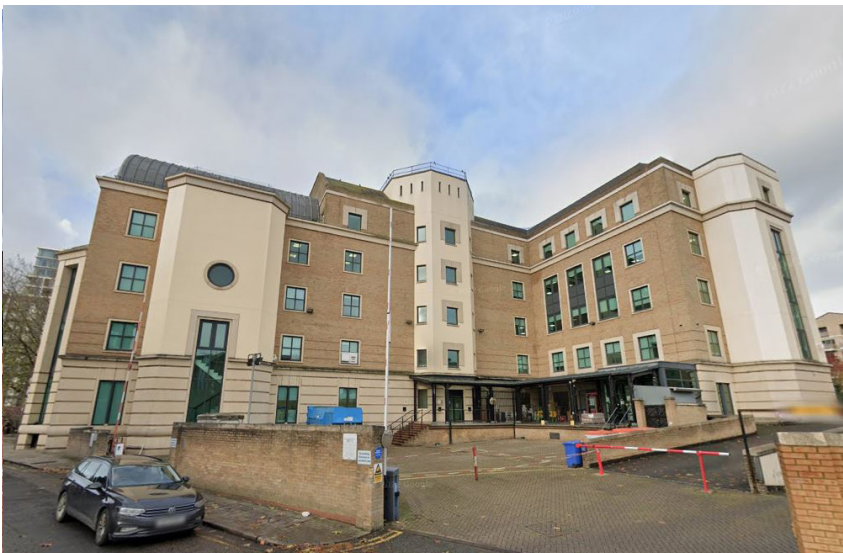
East Elevation – to feature the new windows
