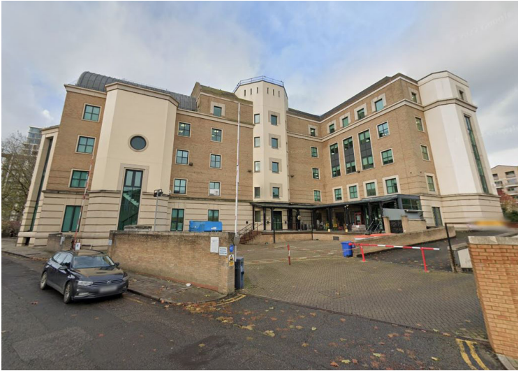
1 - Rear elevation (East) viewed from Gas Works Road
