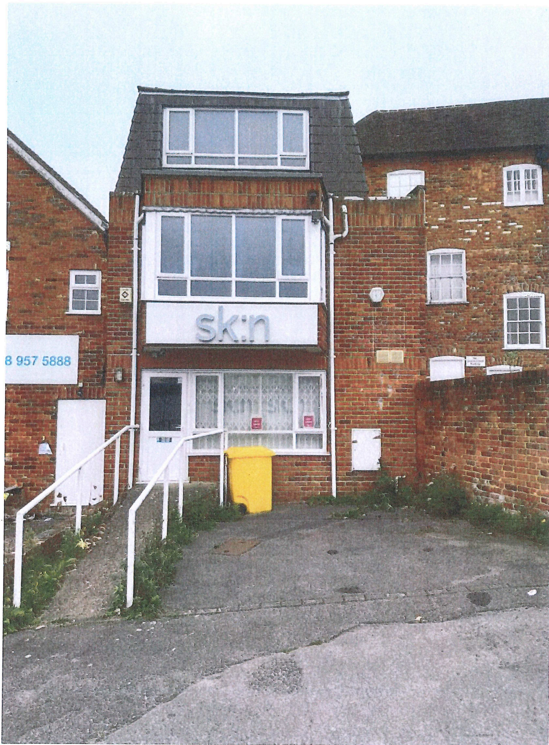
PHOTO - 2 REAR FACADE - EXISTING
