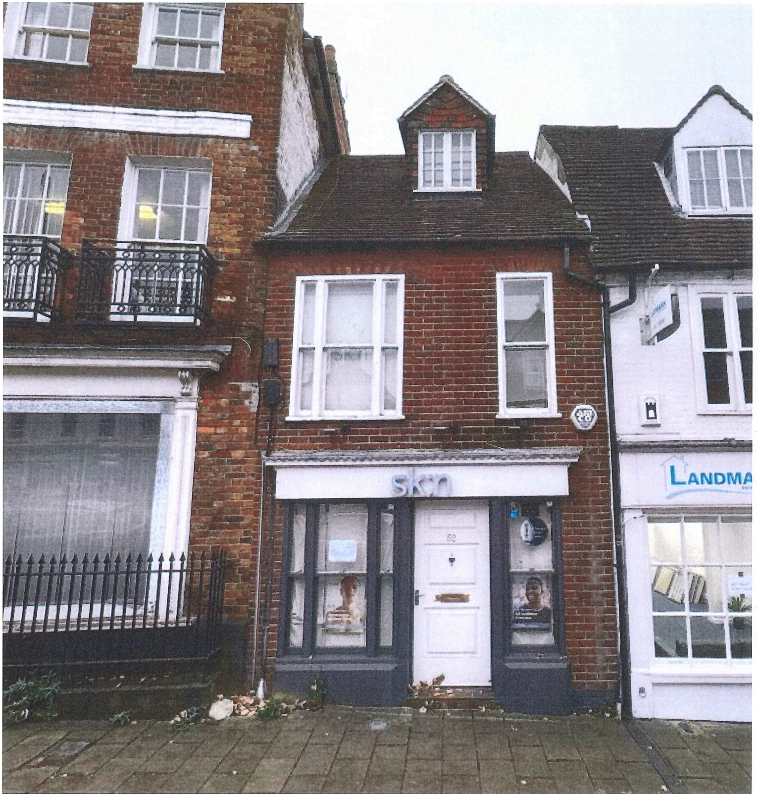
PHOTO - 1 FRONT FACADE - EXISTING
