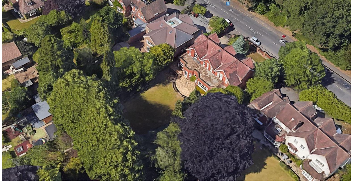
No.50 to North / Northwest; No.42 to South / Southeast of the site
