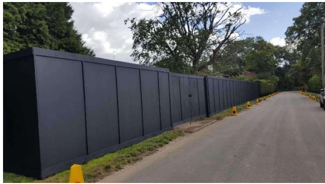
example of solid screens around the construction site
