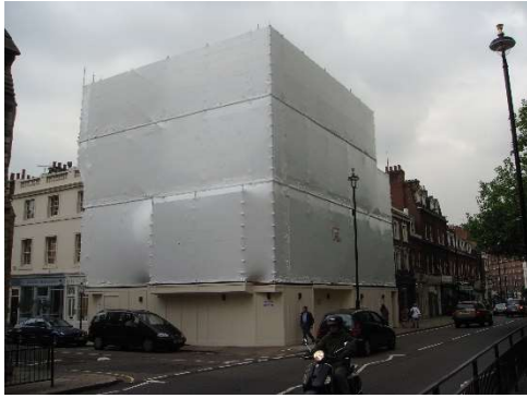
example of screen protected scaffolding
