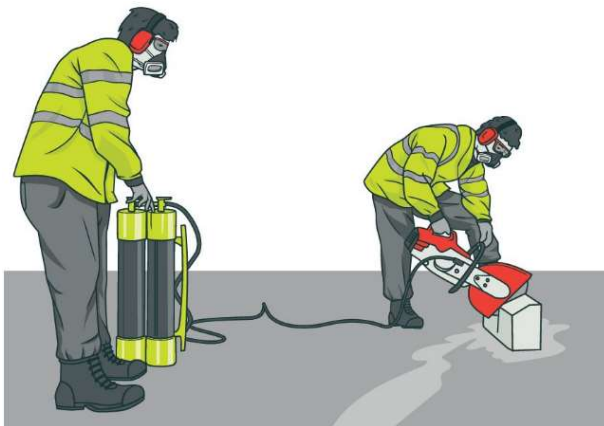
Controlling dust with on-tool water suppression
