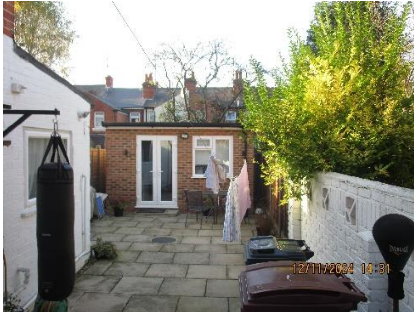
Fig 3: Front View of the existing outbuilding, 12/11/2024
