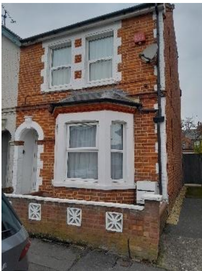
Fig 1: Front View of the property, 13/02/2025
