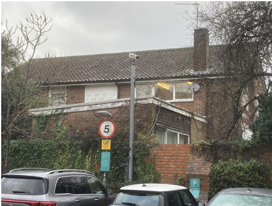
View of the pitched roof from the south, showing the existing clay tiles and chimney. The fascias to one of the two lower roofs are also visible in the foreground
