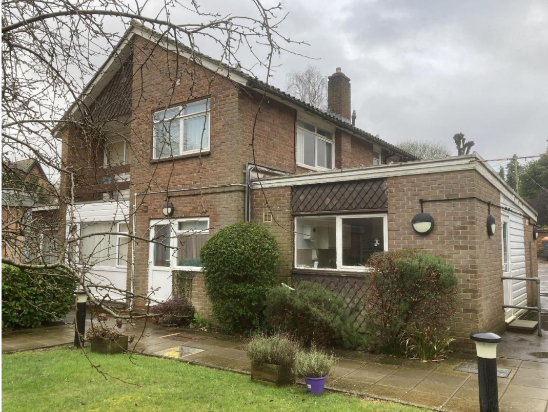
View from the north east, with the fascias to upper and lower level roofs visible, along with the existing chimney to the north elevation
