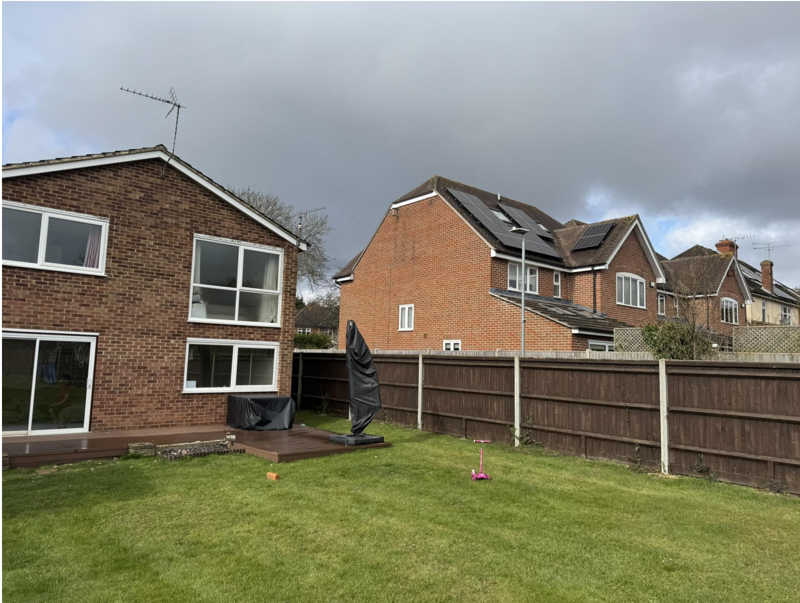
Site Visit Photos taken on 11 March 2025
