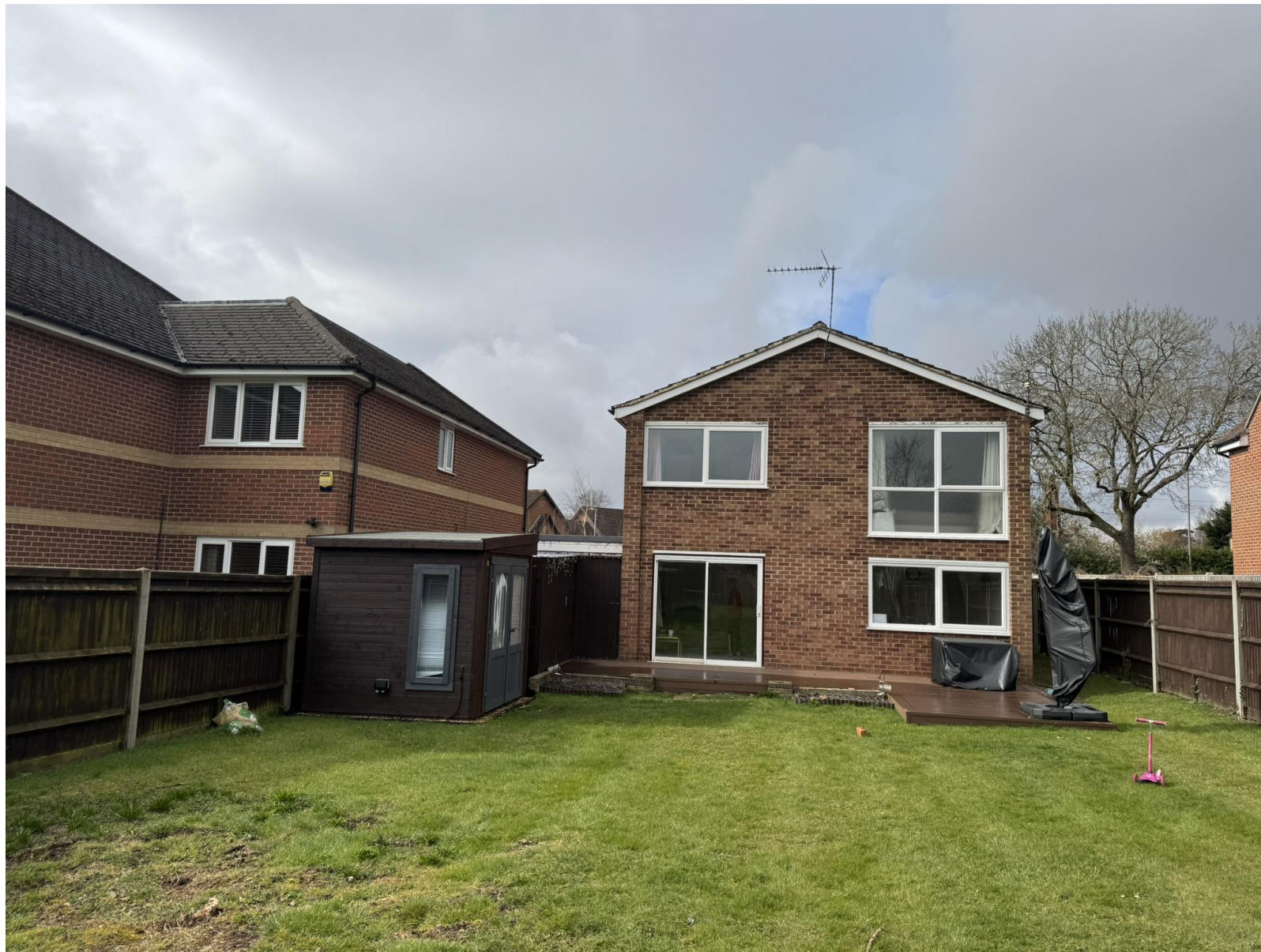
Site Visit Photos taken on 11 March 2025
