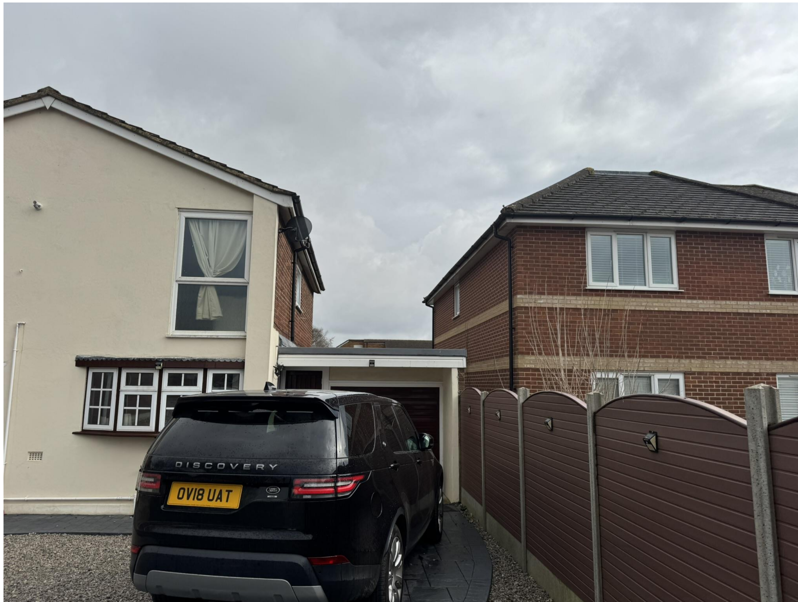
Site Visit Photos taken on 11 March 2025
