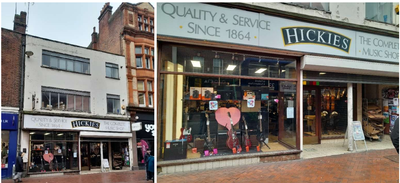
Site photos: existing front elevation looking from Friar Street
