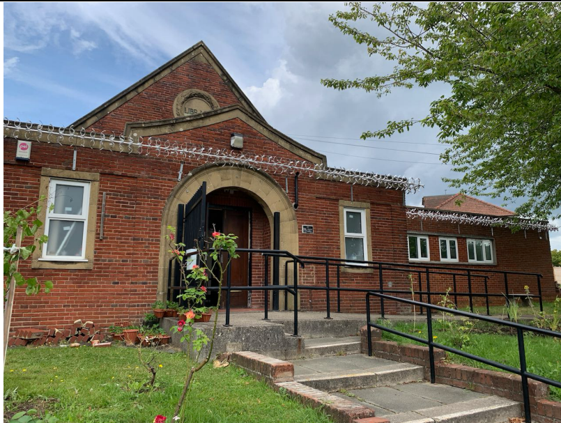
Security fencing around the roof August 2021
