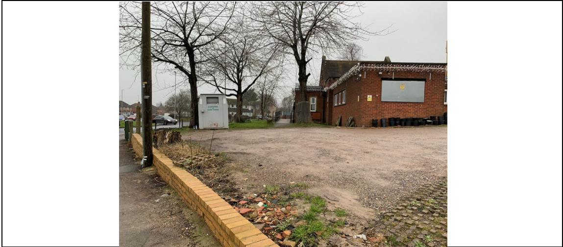
Wall replacing the fence adjacent to the car park (February 2025)
