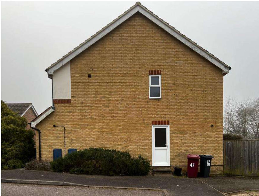
Figure 2 – North-facing facade of 47 Blaenant, the side door and the soft landscape along the property boundary.
