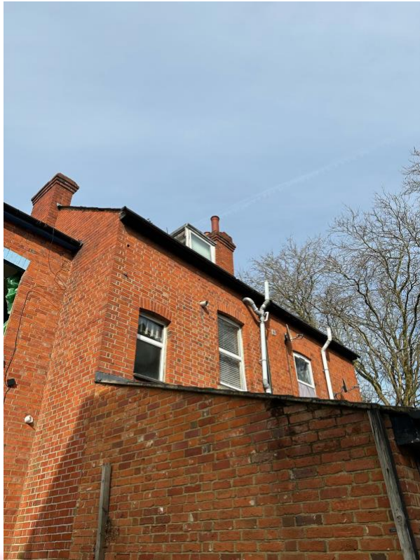
fig 11 Rear Elevation of Terrace example of neighbouring properties
