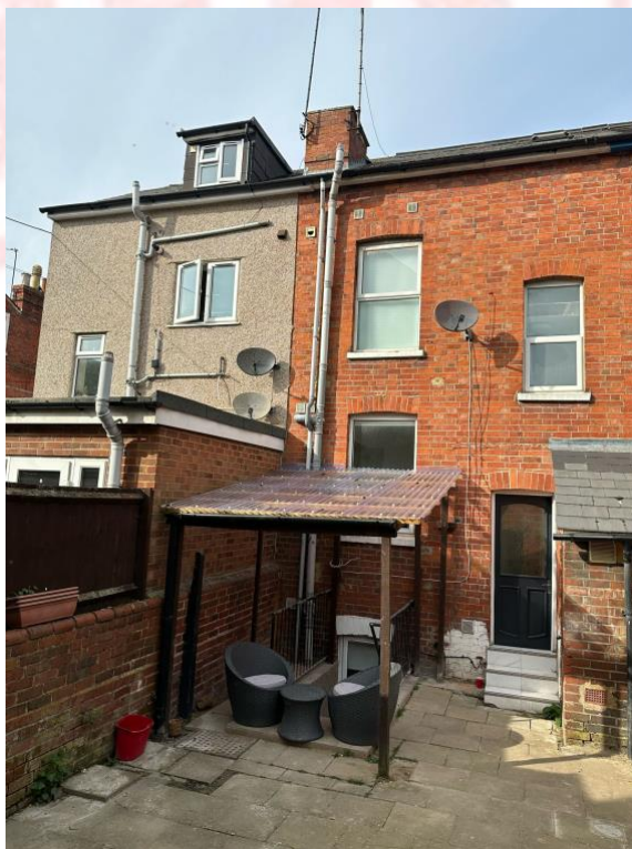
fig 10 Rear Elevation of Terrace example of neighbouring properties
