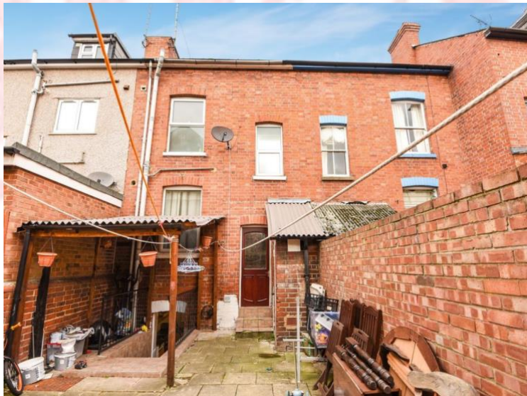
fig 12 Rear Elevation Prior to works
