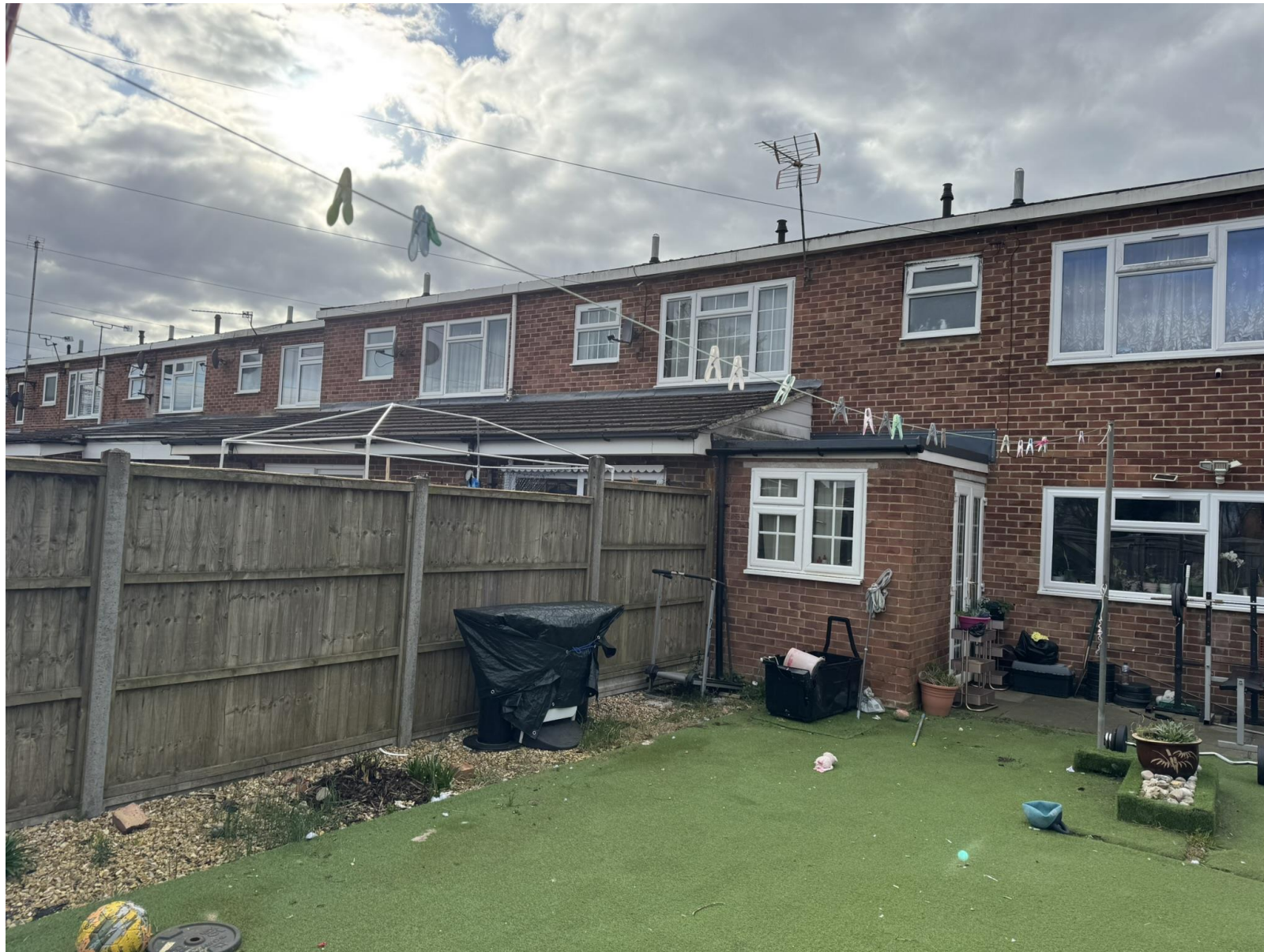
Site Visit Photos taken on 11 March 2025
