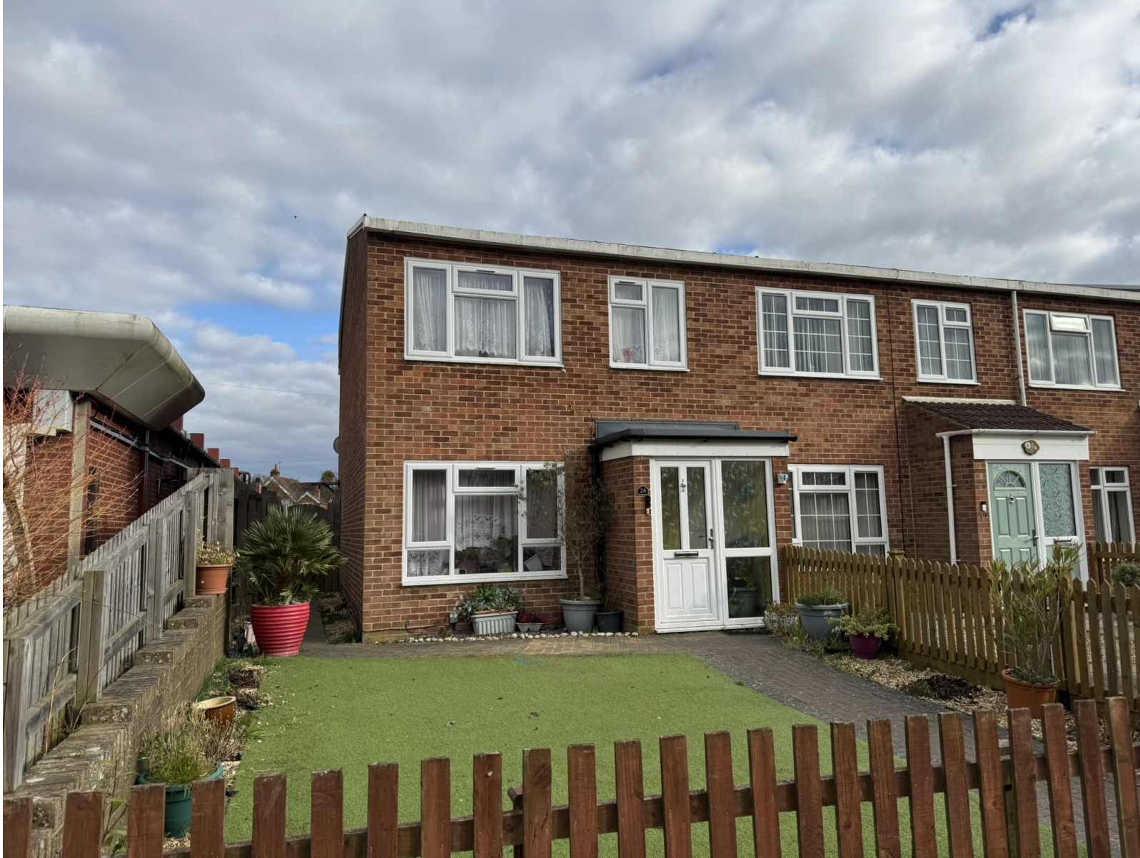
Site Visit Photos taken on 11 March 2025
