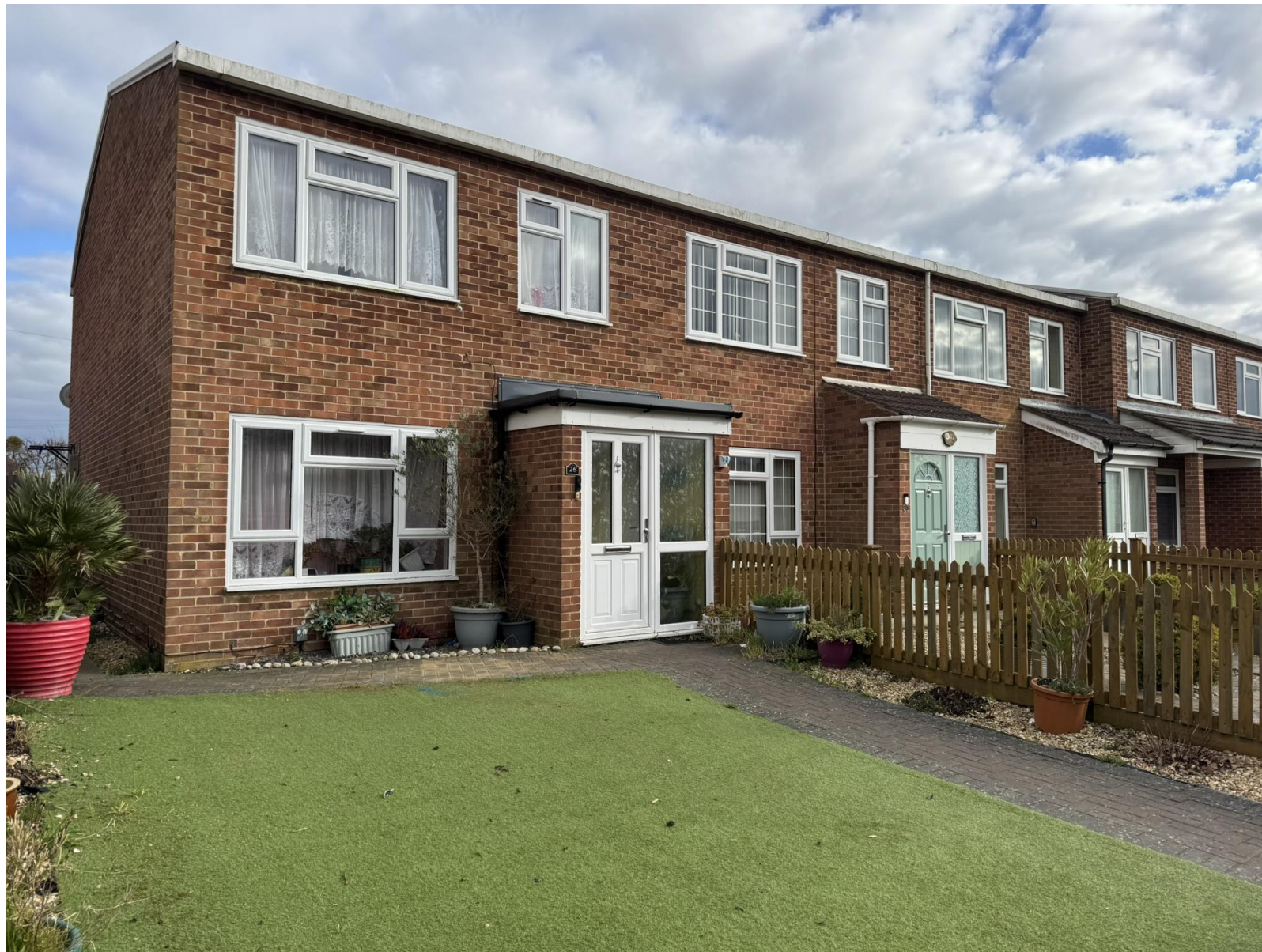
Site Visit Photos taken on 11 March 2025
