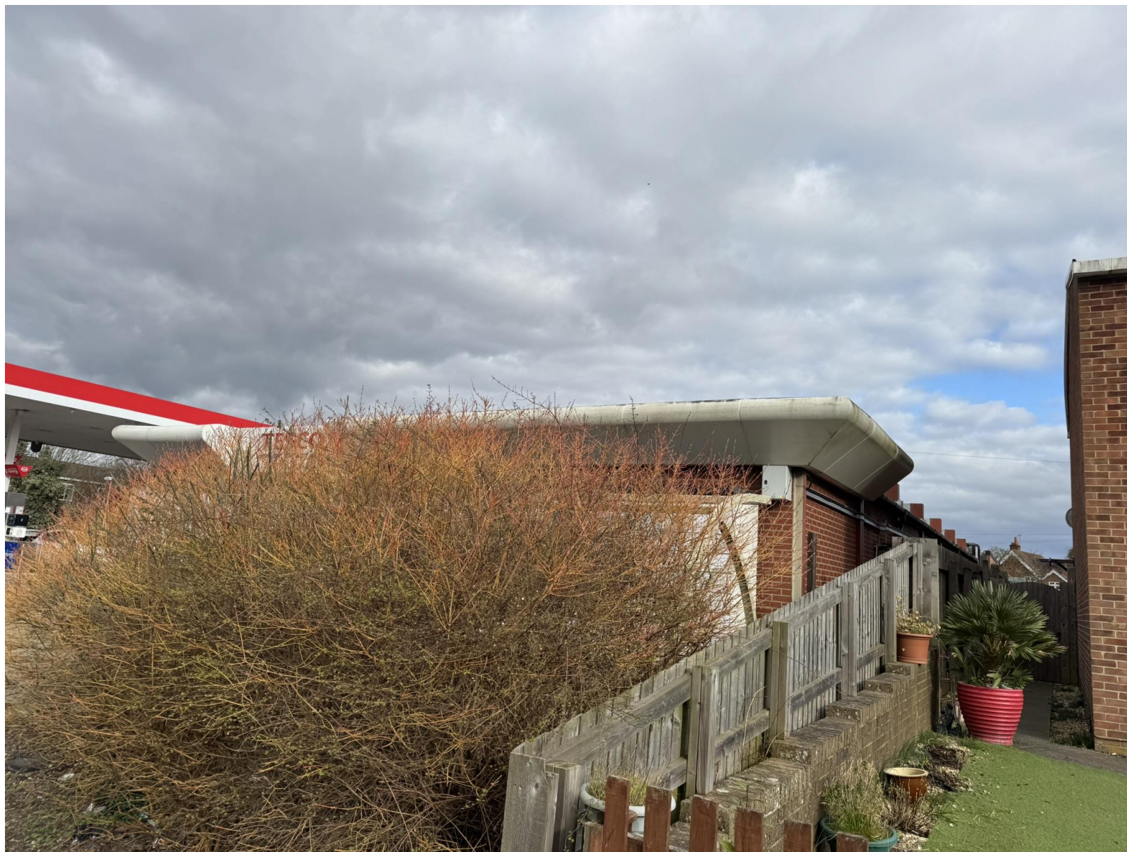
Site Visit Photos taken on 11 March 2025
