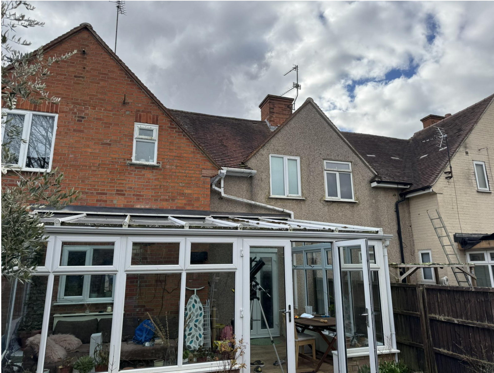
Site Visit Photos taken on 11 March 2025
