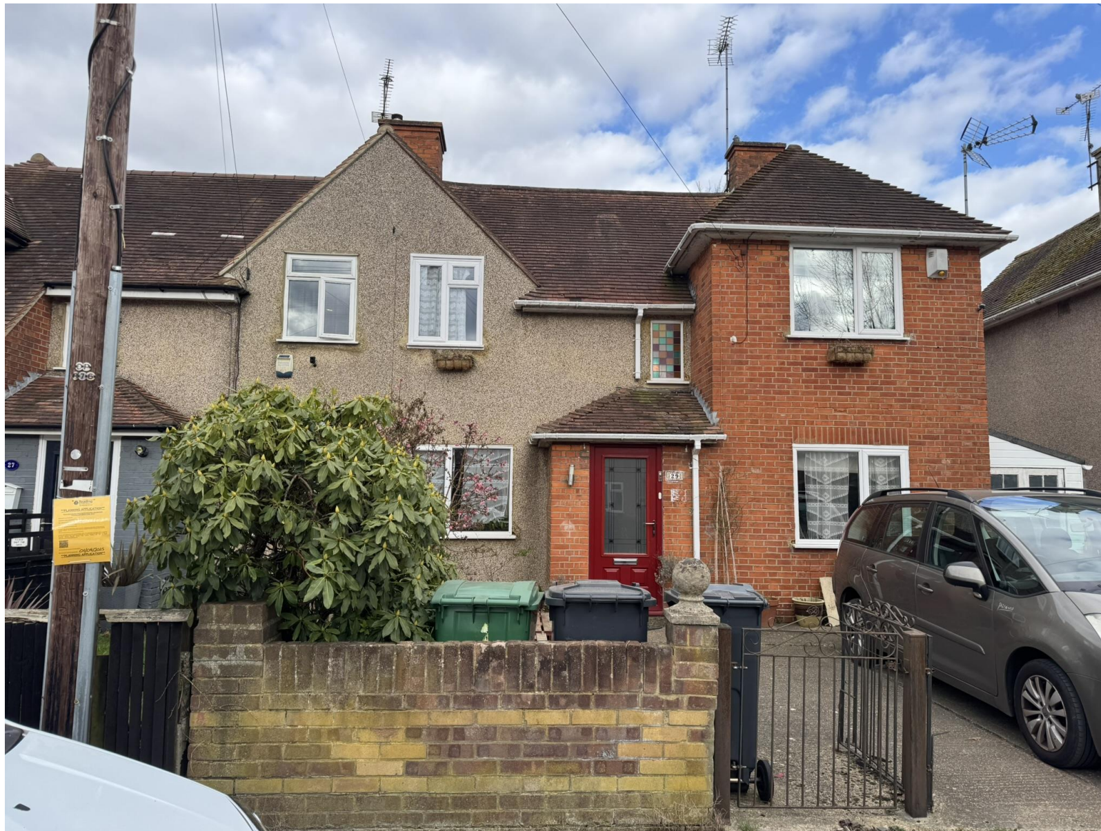
Site Visit Photos taken on 11 March 2025
