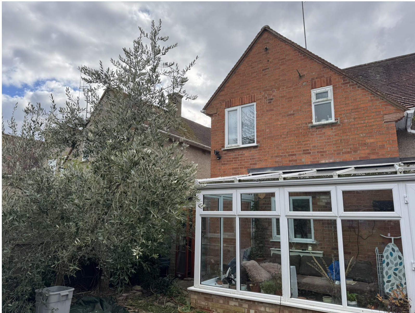
Site Visit Photos taken on 11 March 2025
