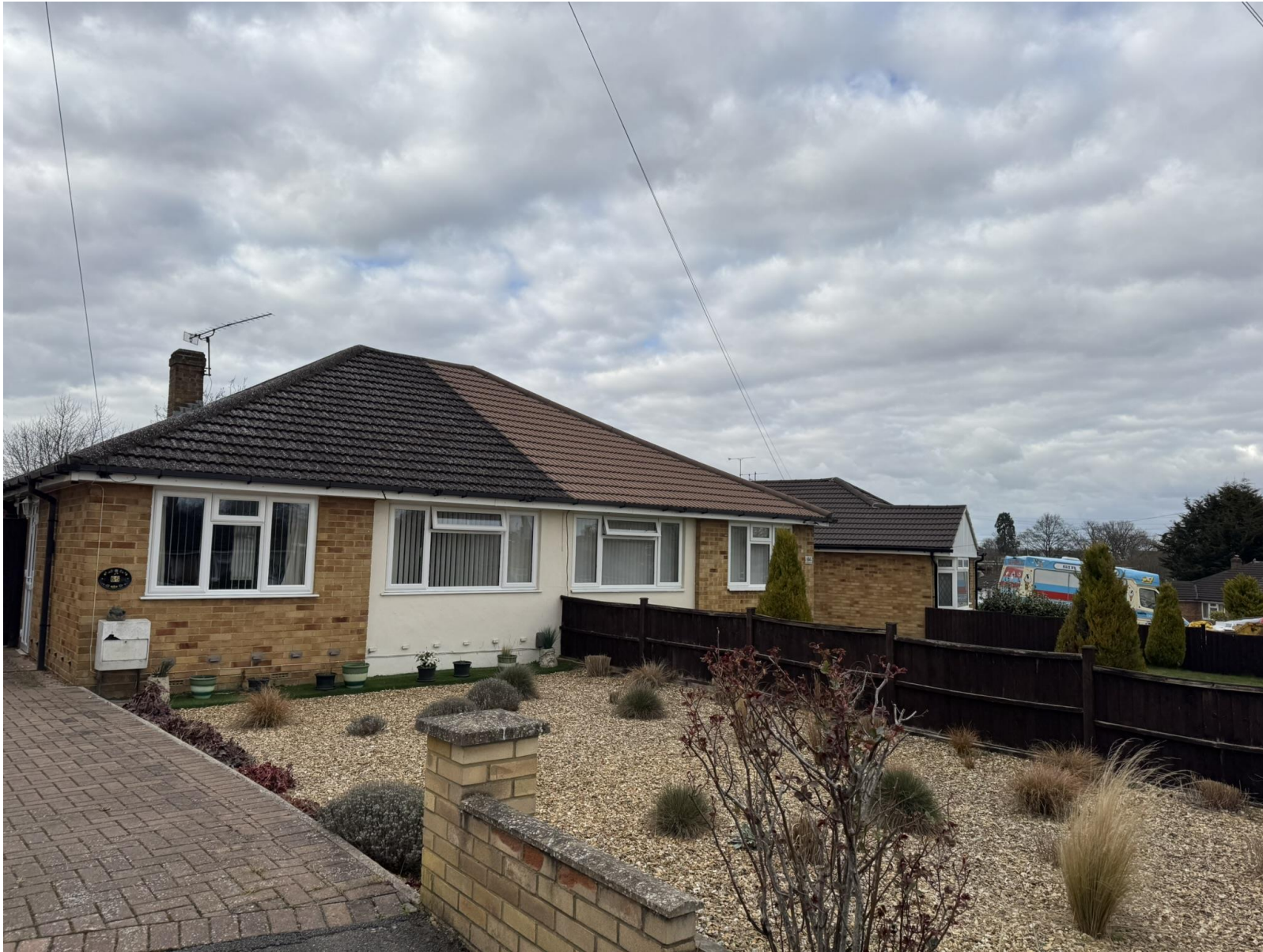
Site Visit Photos taken on 11 March 2025
