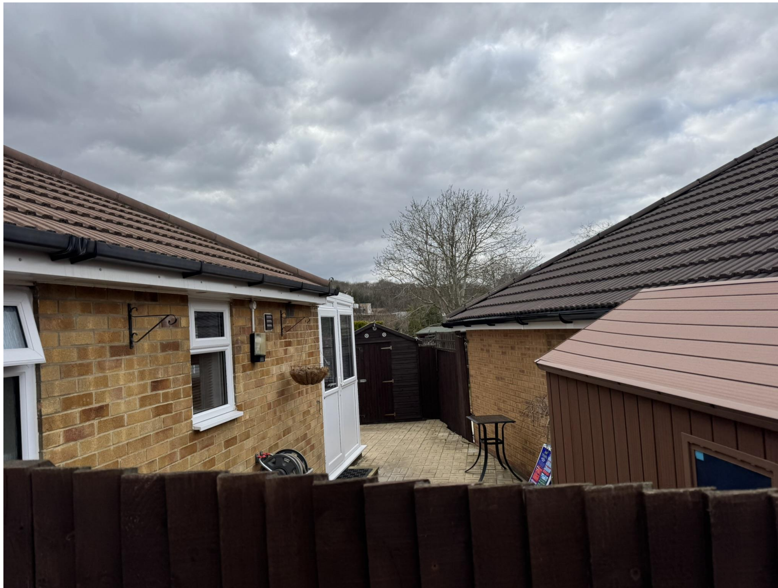
Site Visit Photos taken on 11 March 2025
