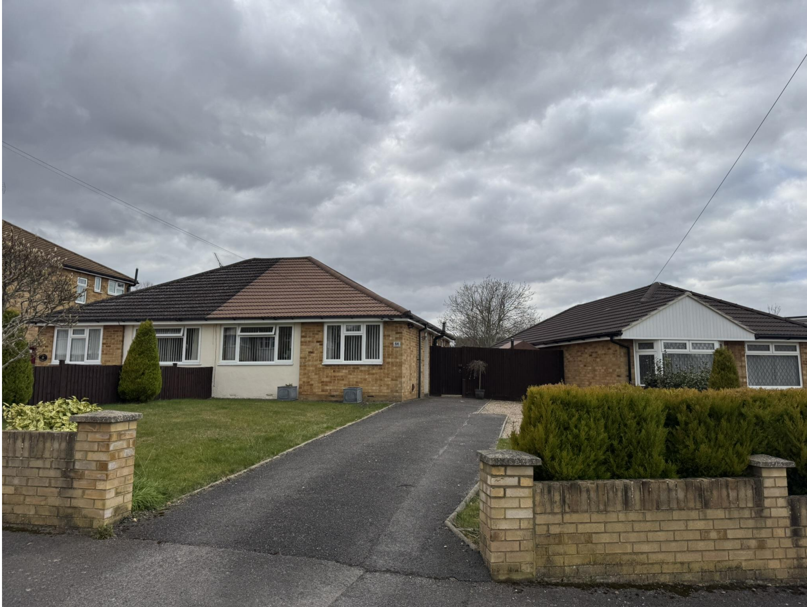
Site Visit Photos taken on 11 March 2025
