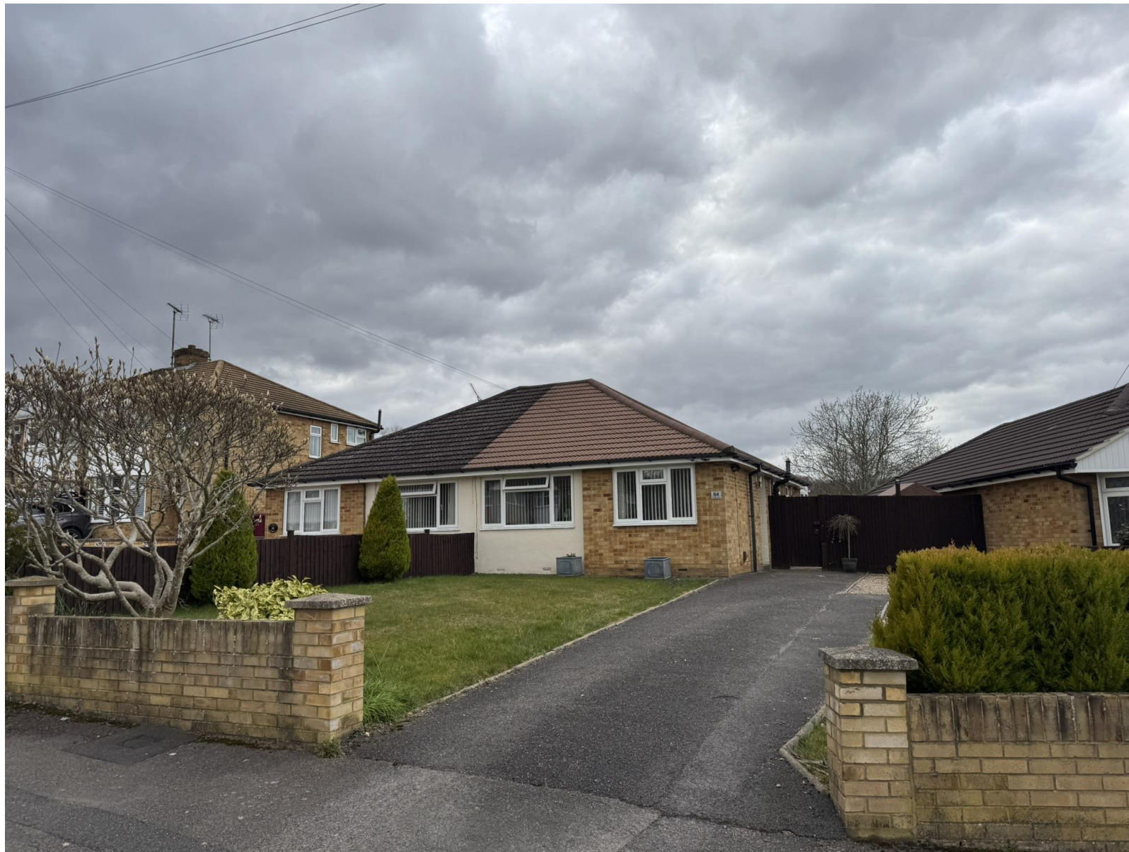
Site Visit Photos taken on 11 March 2025
