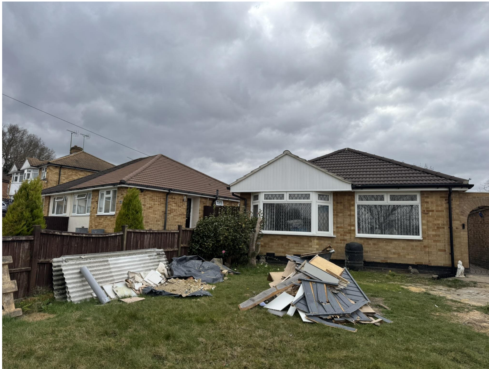
Site Visit Photos taken on 11 March 2025
