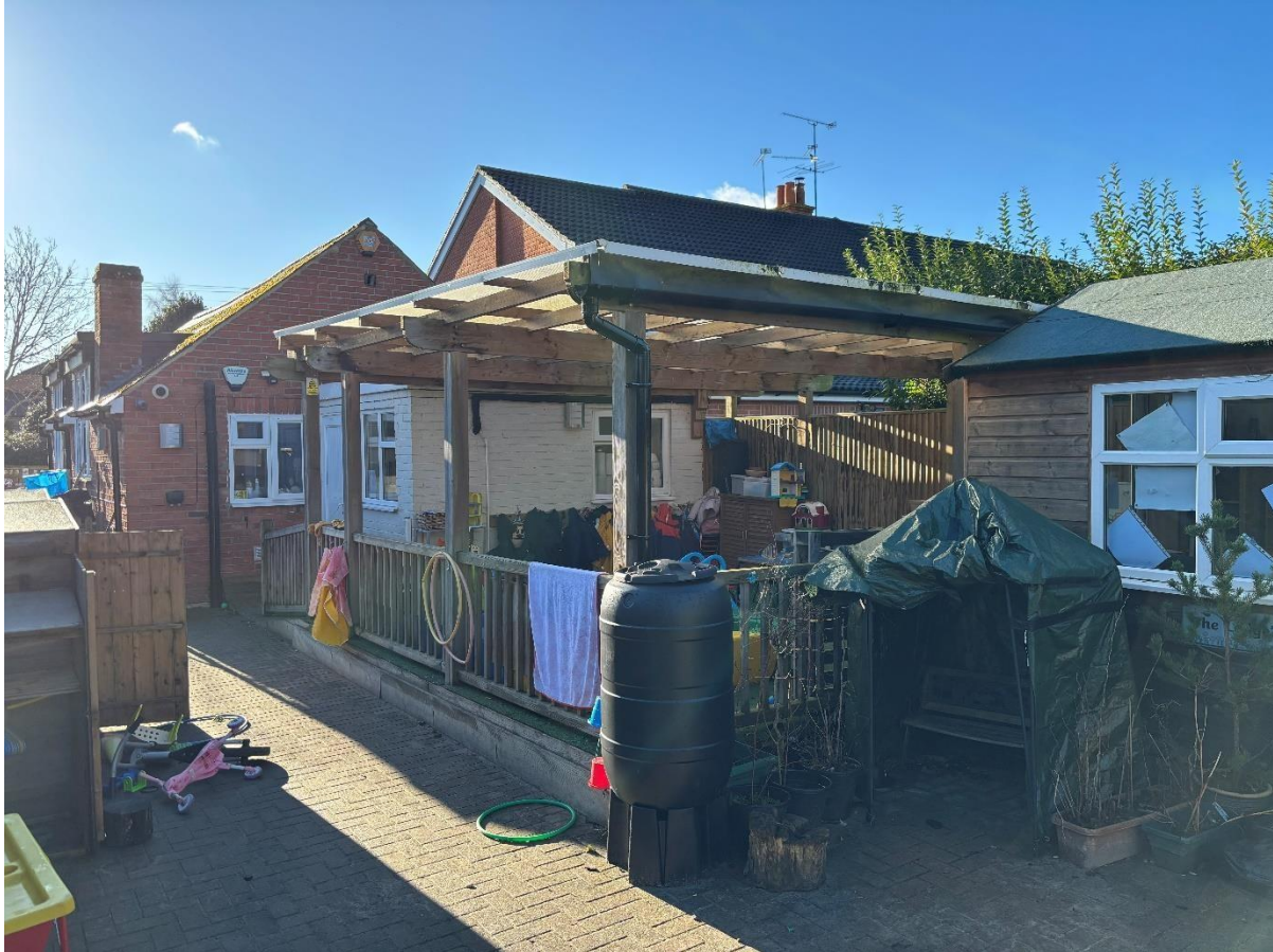
Rear of building showing covered play area/outdoor classroom
