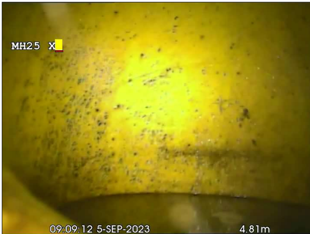
Photo: 349_3a, 00:00:00 4.8m, Manhole Remark:MH
