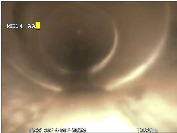
Photo: 204_4a, 00:00:00 11m, Junction at 10 o'clock, dia 150 mm
