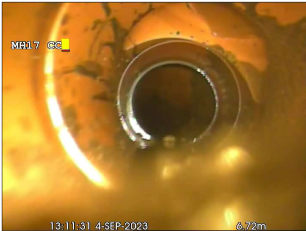
Photo: 260_6a, 00:00:00 6.8m, Junction at 01 o'clock, dia 100 mm
