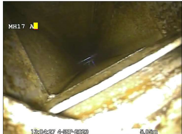
Photo: 231_7a, 00:00:00 5.85m, Finish Survey, Remark: DP
