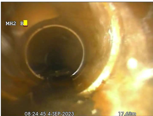
Photo: 3_6a, 00:00:00 17.8m, Junction at 12 o'clock, dia 80 mm
