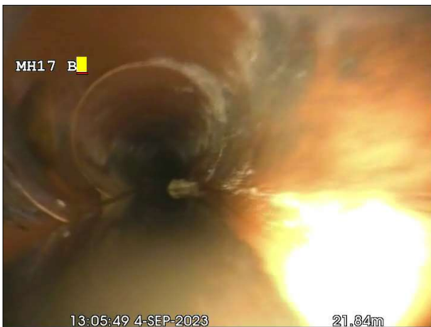
Photo: 247_10a, 00:00:00 22m, Junction at 10 o'clock, dia 150 mm
