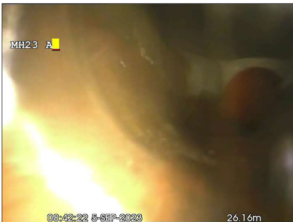
Photo: 314_11a, 00:00:00 26.2m, Manhole Remark: MH
