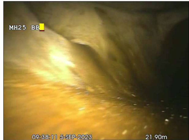
Photo: 363_7a, 00:00:00 21.9m, Manhole Remark: MH
