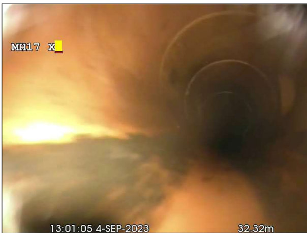
Photo: 234_6a, 00:00:00 33m, Junction at 03 o'clock, dia 100 mm
