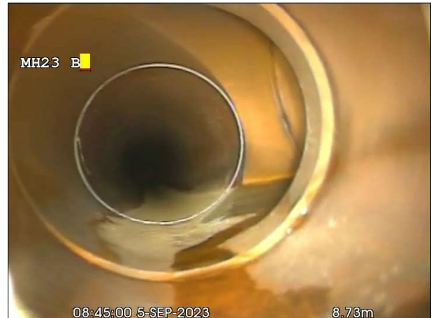
Photo: 321_5a, 00:00:00 8.9m, Junction at 02 o'clock, dia 100 mm
