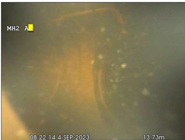
Photo: 36_9a, 00:00:00 13.7m, Manhole Remark: Chamber visible
