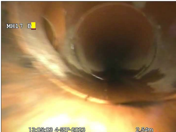
Photo: 240_3a, 00:00:00 2.7m, Junction at 11 o'clock, dia 150 mm
