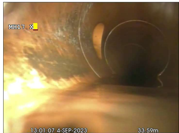
Photo: 236_8a, 00:00:00 34m, Junction at 10 o'clock, dia 100 mm
