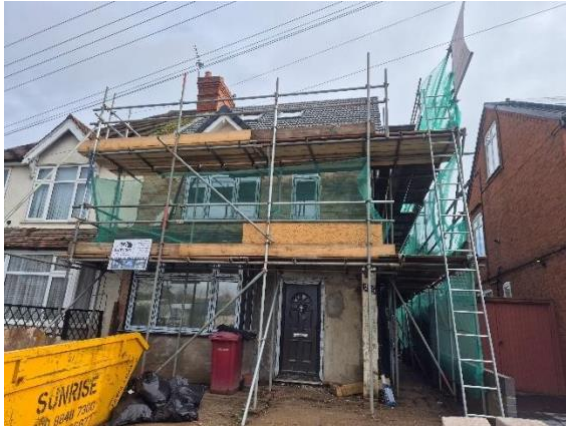
Photograph 1: Western elevation of B1.
