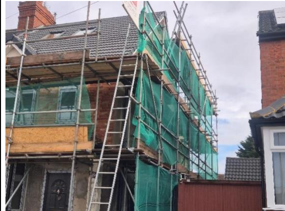
Photograph 2: Southern elevation of B1.
