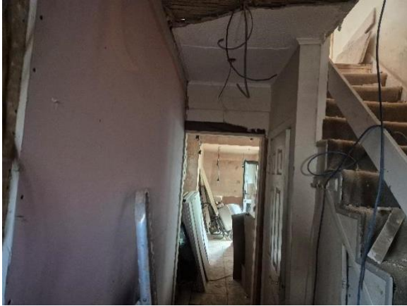
Photograph 8: Interior of B1.
