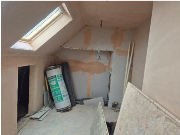
Photograph 6: Converted loft of B1.
