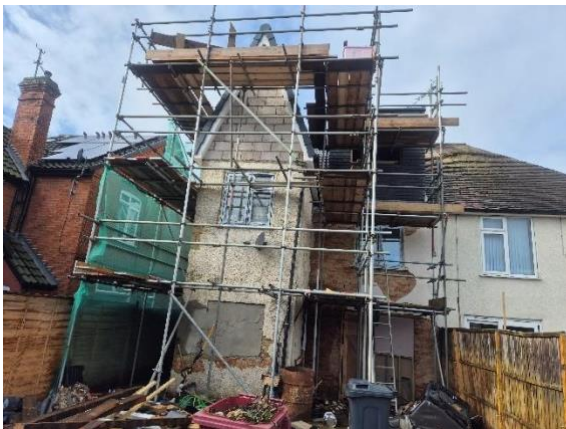
Photograph 3: Eastern elevation of B1.
