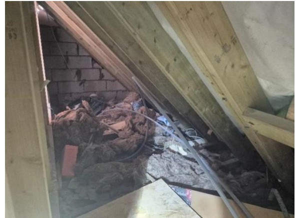
Photograph 7: Eaves void on the western side of B1.
