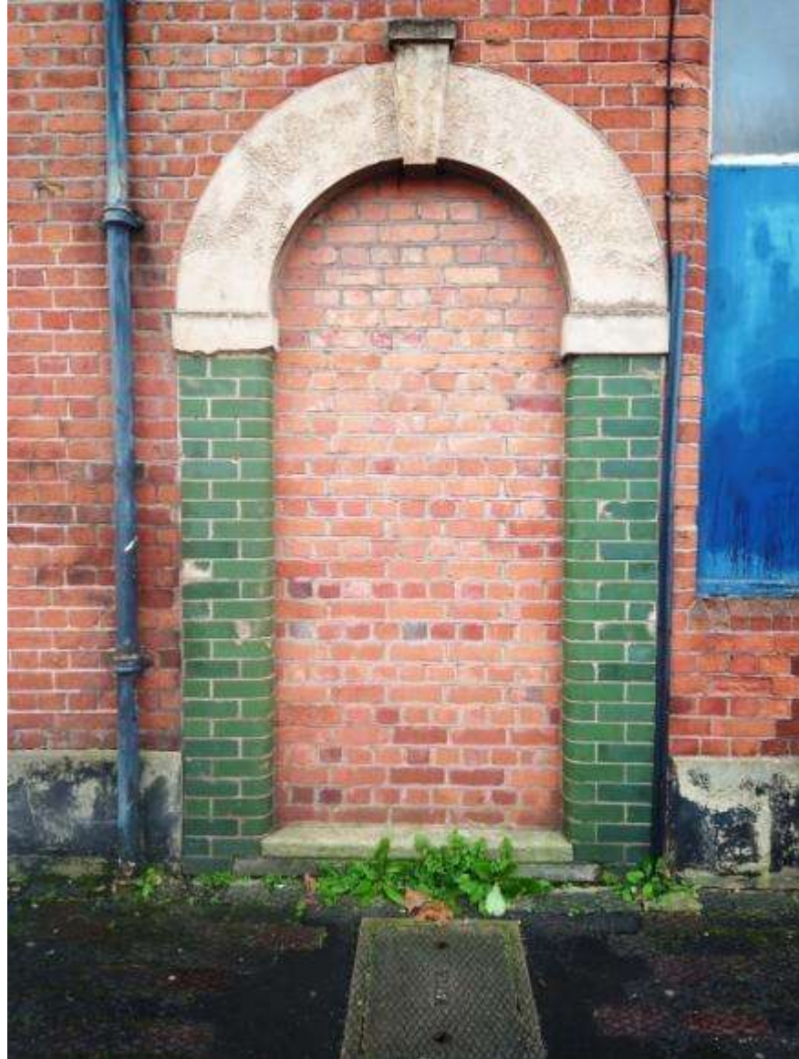
Fig 3.3.4: Closed-up door opening
