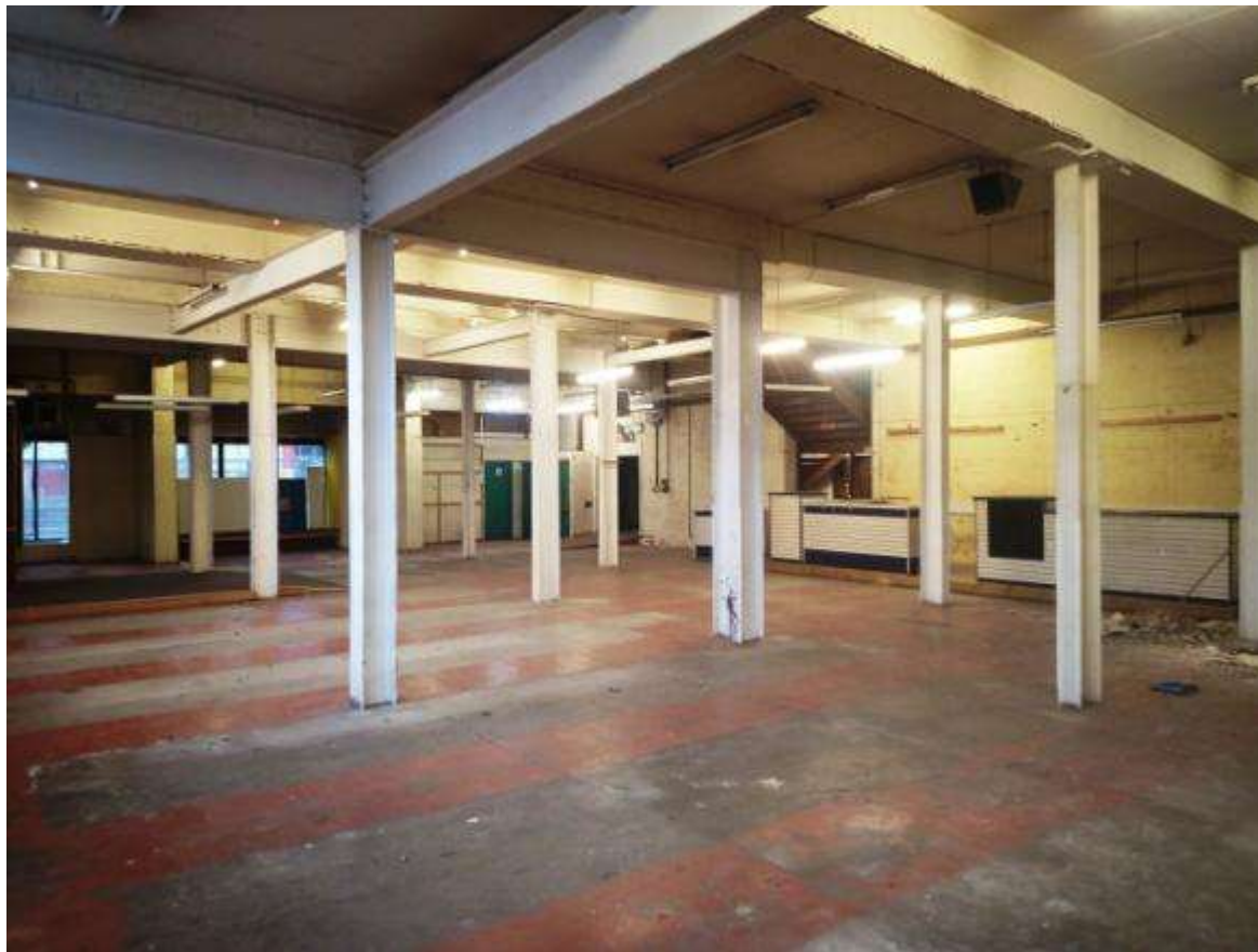
Fig 4.1: North block ground floor looking from back to front
