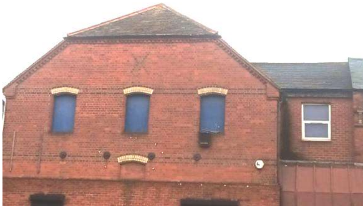
Fig 3.3.12: Upper east gable to N° 71
