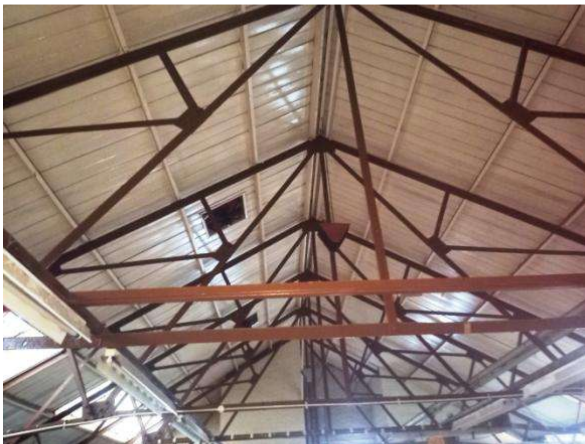
Fig 4.4.4: Roof trusses to north block man roof
