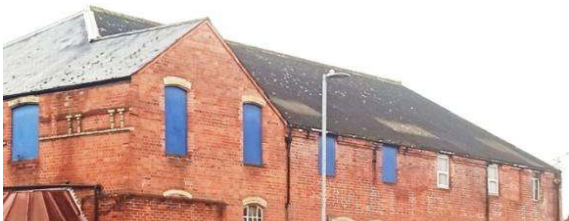
Fig 3.1.1: Roof to north block (73)
