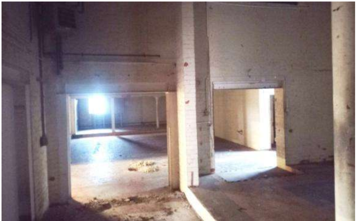
Fig 4.3.6: Dividing wall between front and rear section of south block
