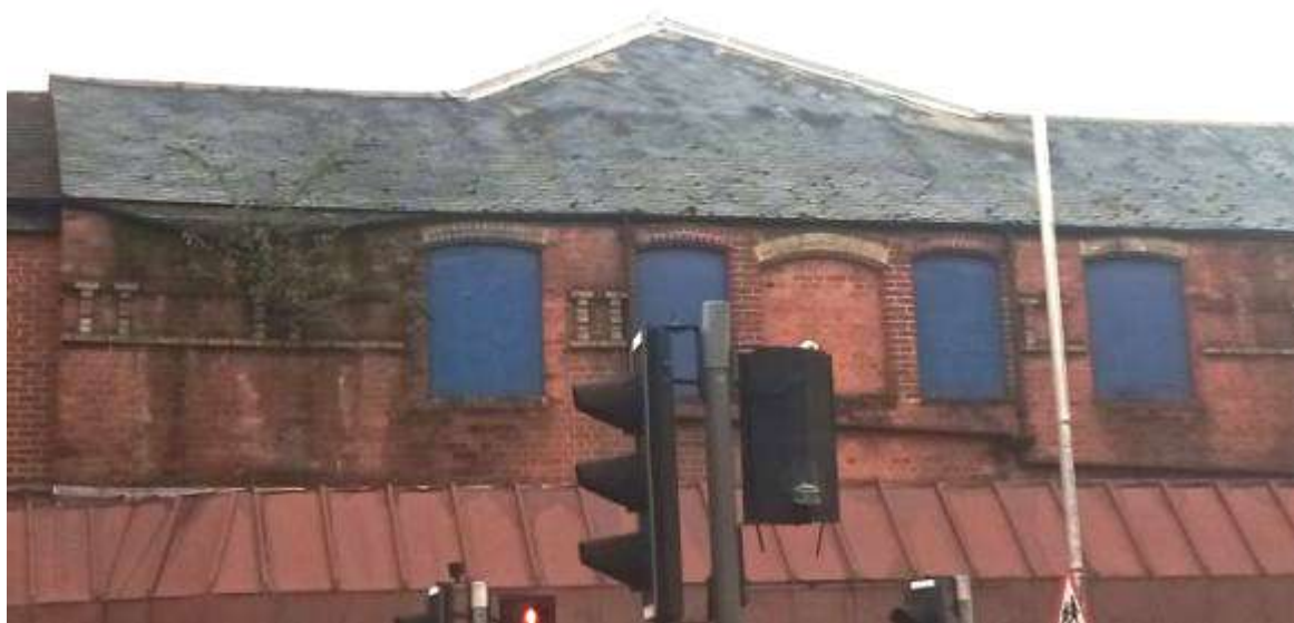
Fig 3.3.9: First floor front windows
