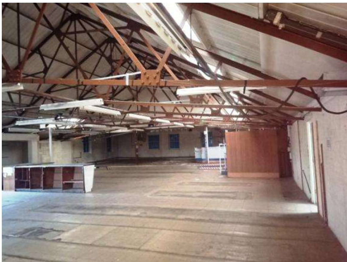
Fig 4.4: North block first floor looking towards the front
