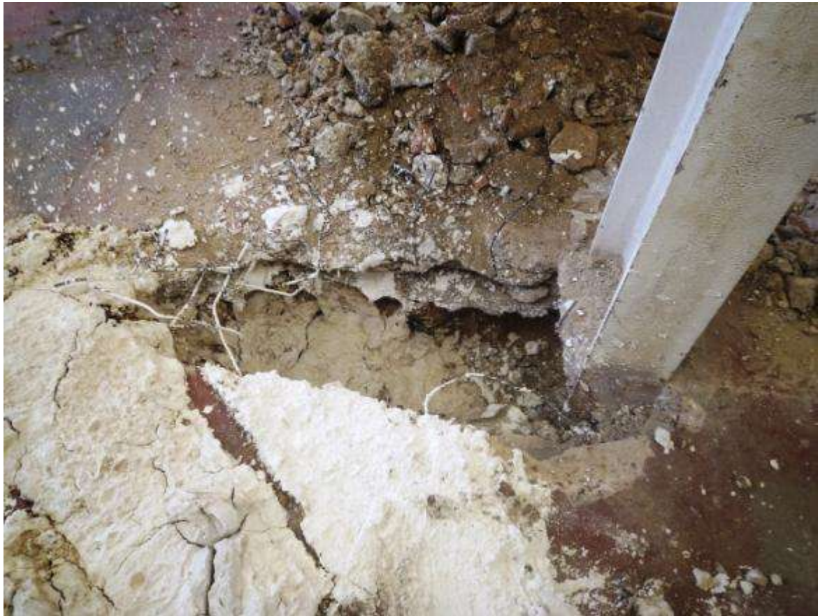
Fig 4.1.5: Column with opened-up floor
