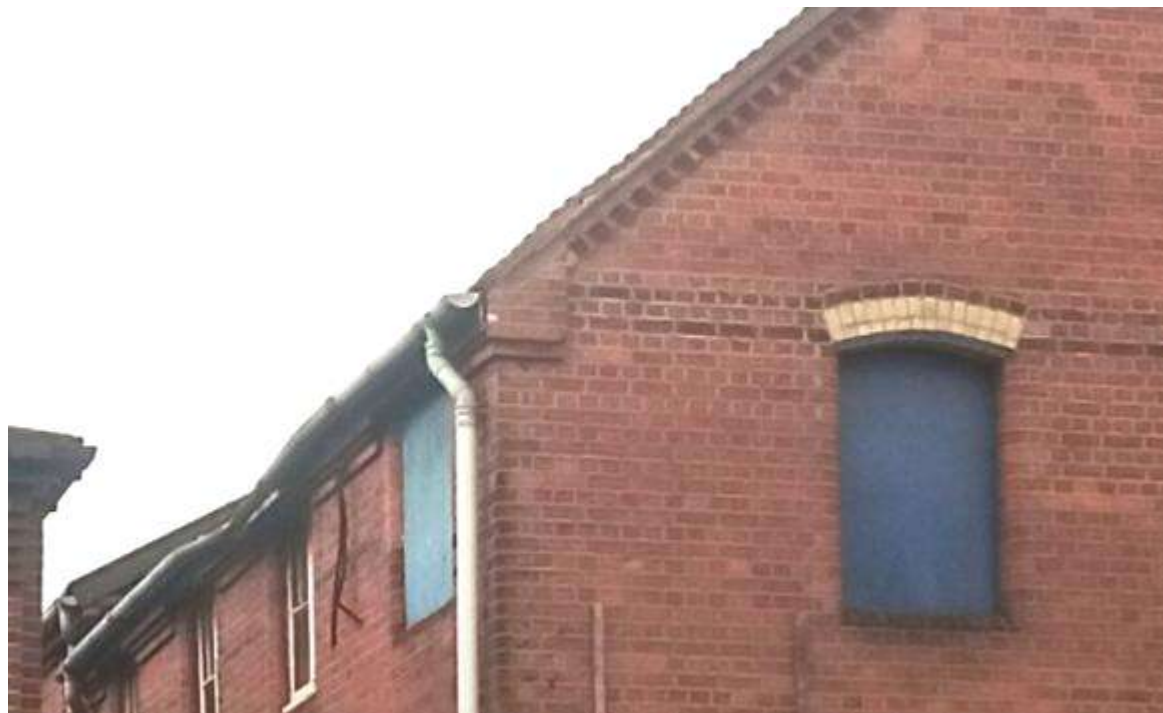
Fig 3.2.1: East verge and south wall eaves
