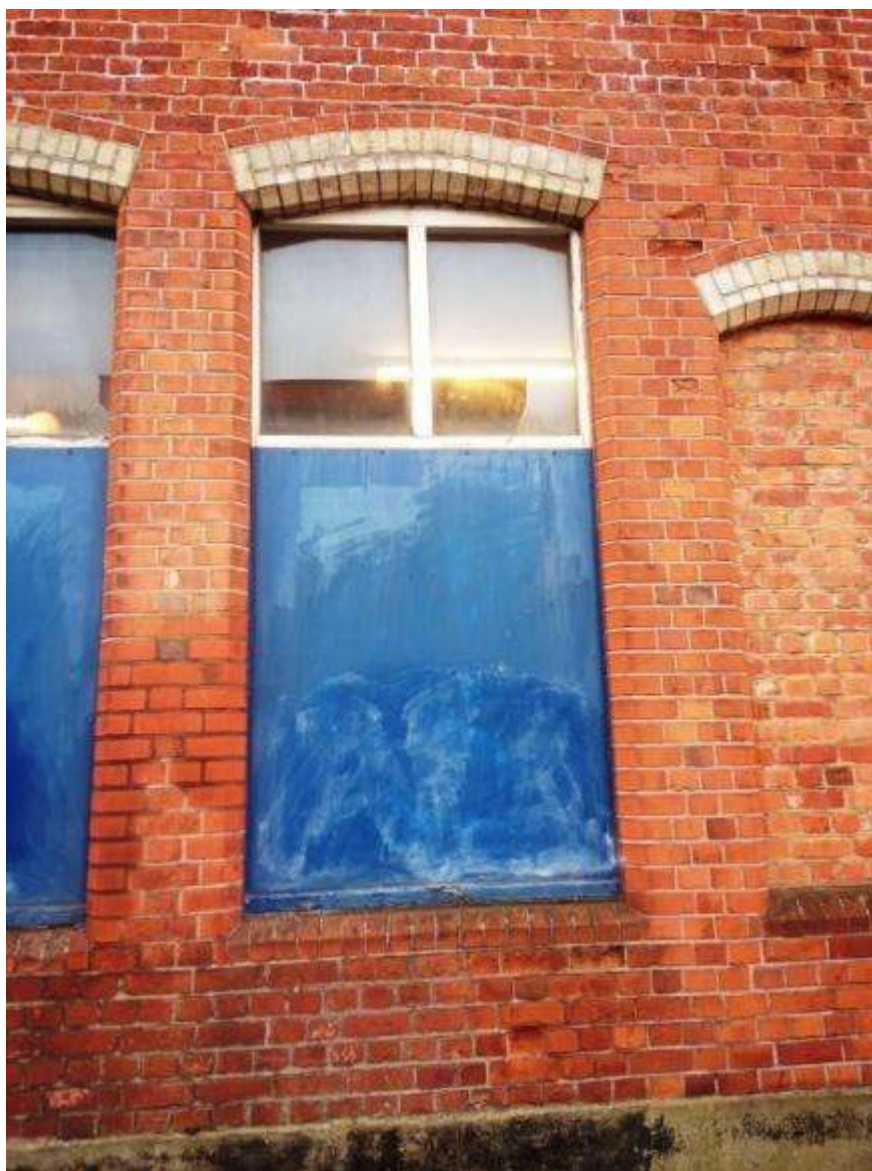
Fig 3.3.2: Ground floor north windows
