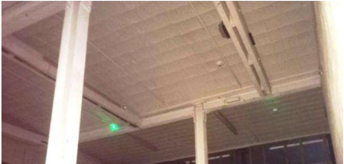
Fig 4.3.5: Underside of brick upper floor
