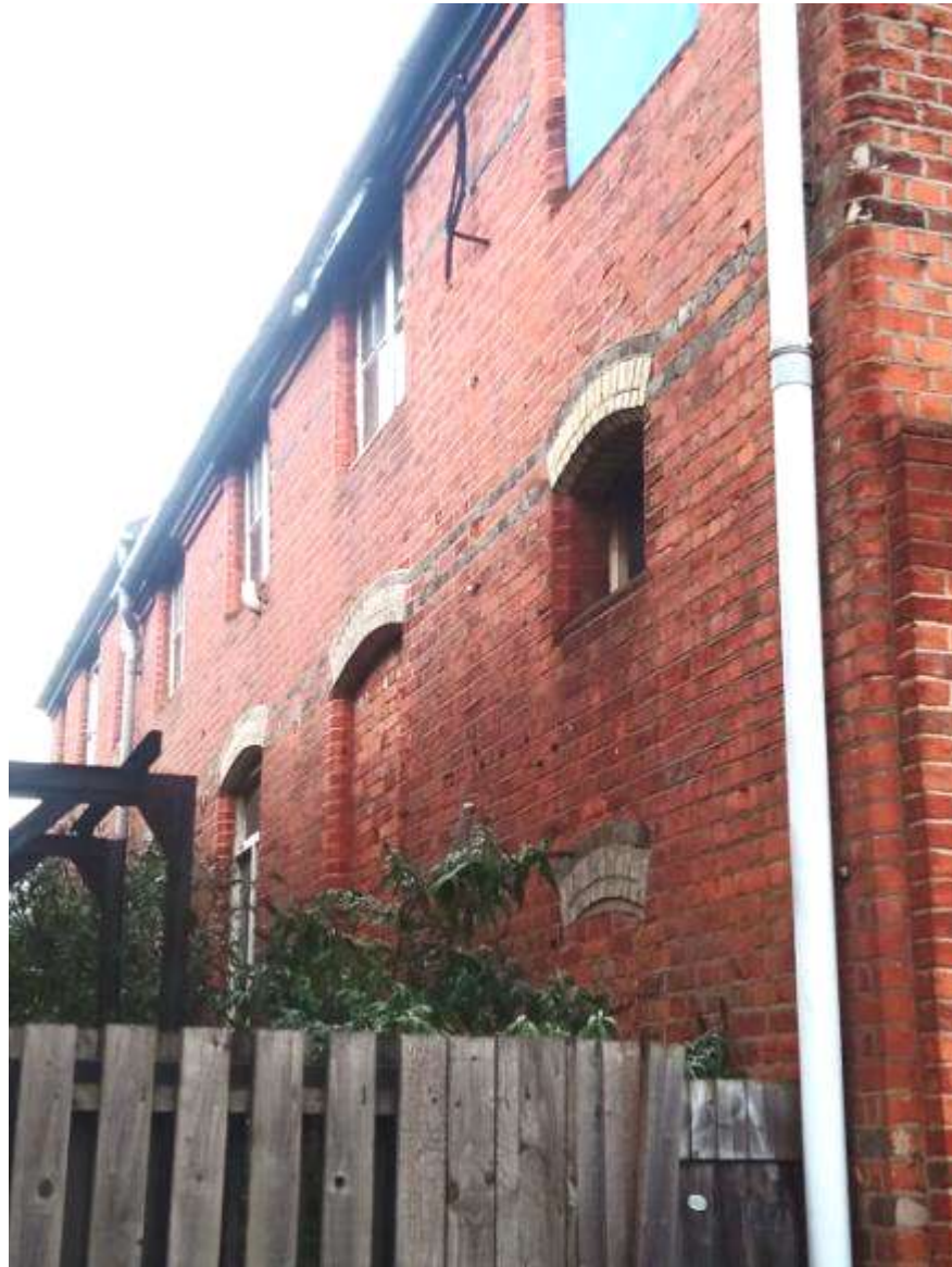
Fig 3.3.17: Restricted view of south elevation, showing eaves level change
