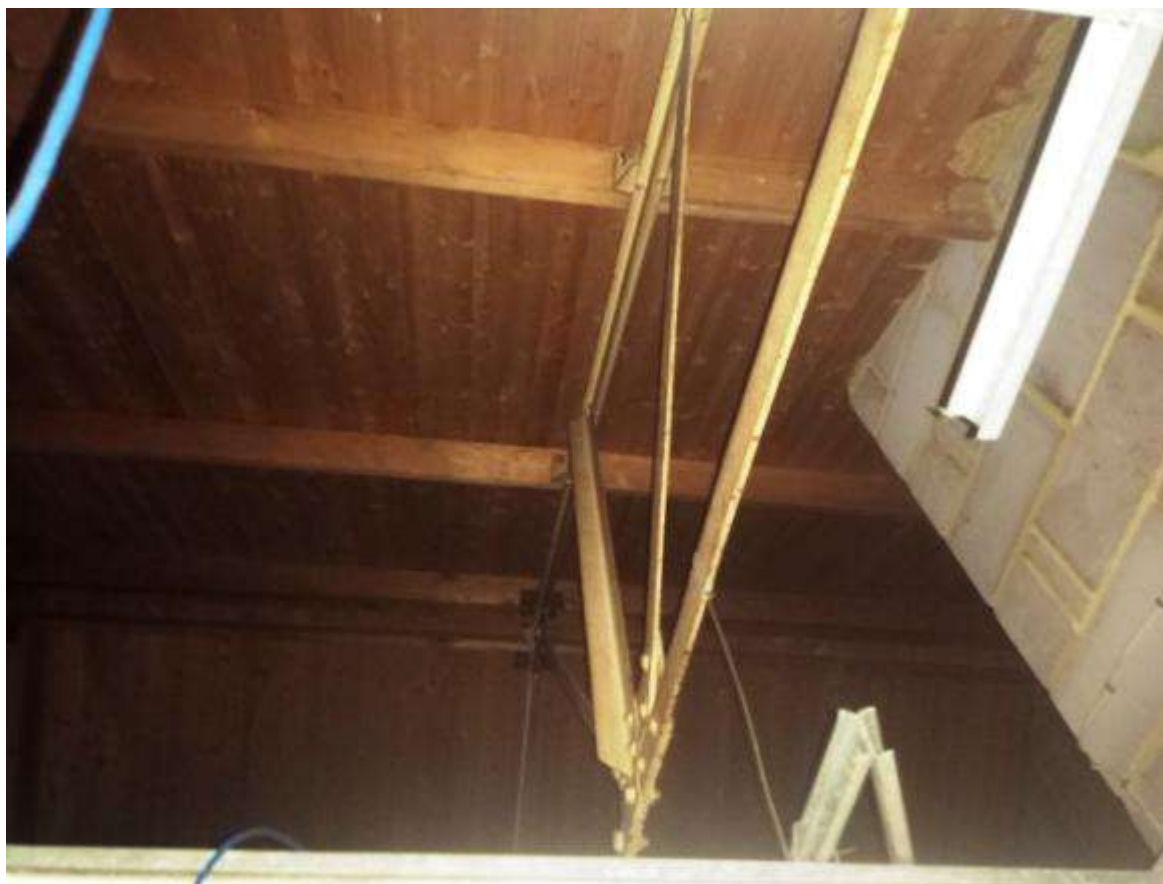
Fig 4.6.7: South block roof truss at west end above suspended ceiling
