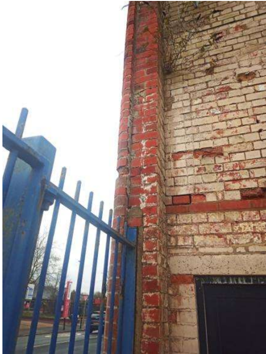
Fig 3.3.21: Link nib on northwest corner to removed building
