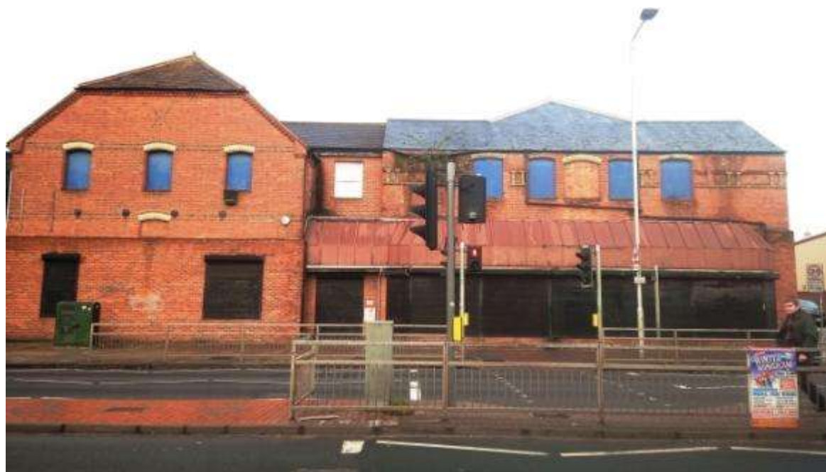
Fig 2.2.5: Front cross range to N° 73 (left) and new infill against south block (71)
