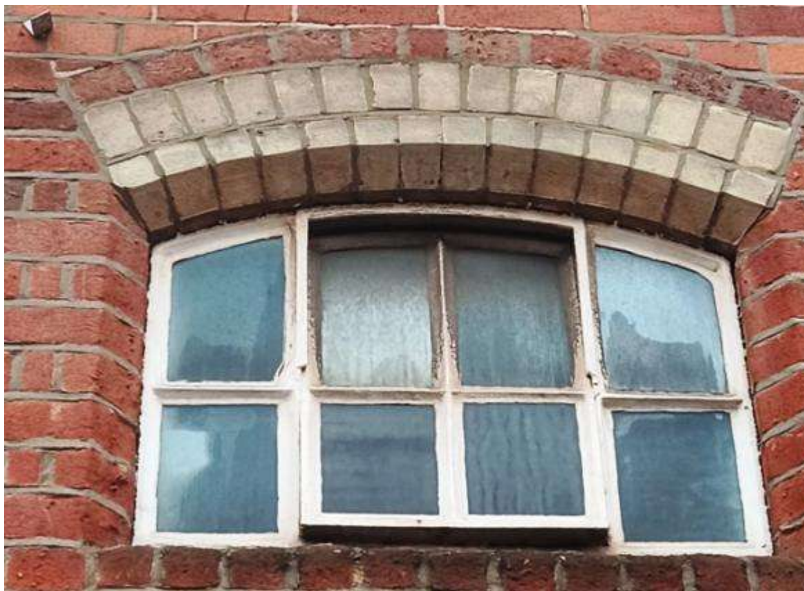
Fig 3.4.2: Cast iron window
