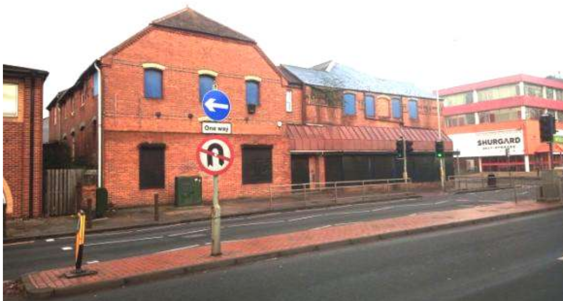
Fig 2.1.1: 71 – 73 Caversham Road from the southeast (71 left)
