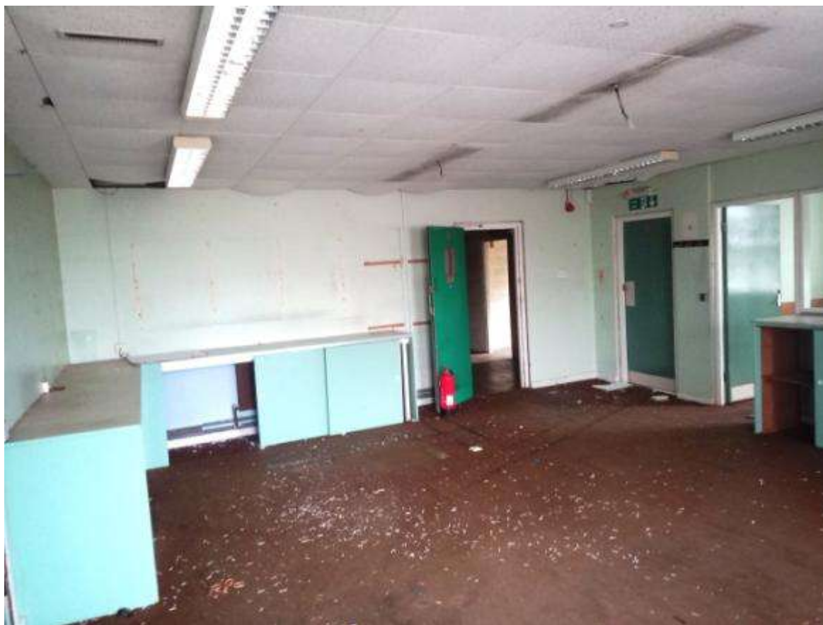
Fig 4.6.3: South block first floor west end office
