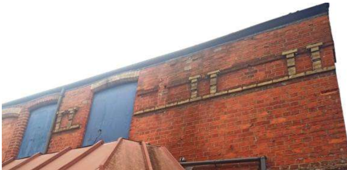
Fig 3.3.10: Decorative brickwork to front of 73.
