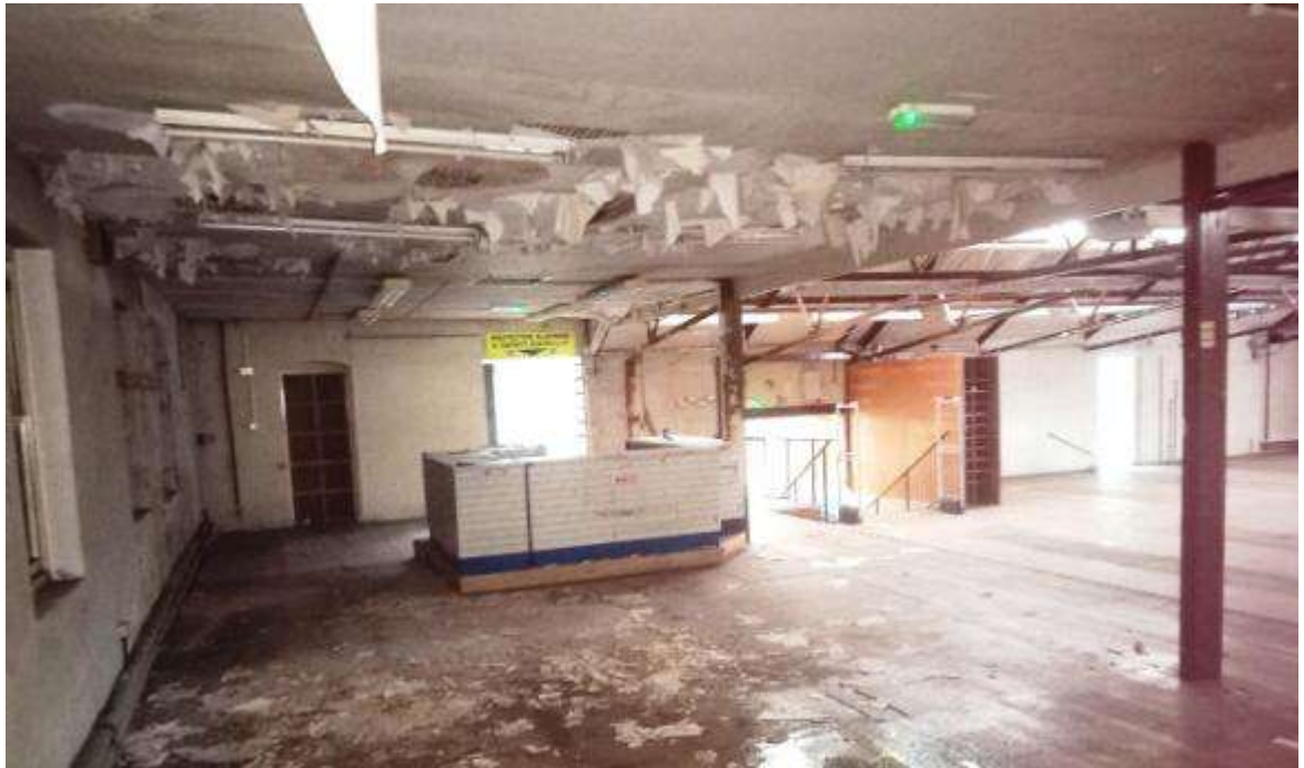
Fig 4.4.6: Lower ceiling to former office area to front of first floor north block (73
