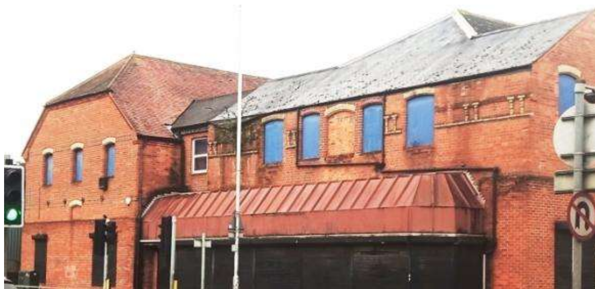
Fig 3.1.7: Front roofs with low level zinc roof
