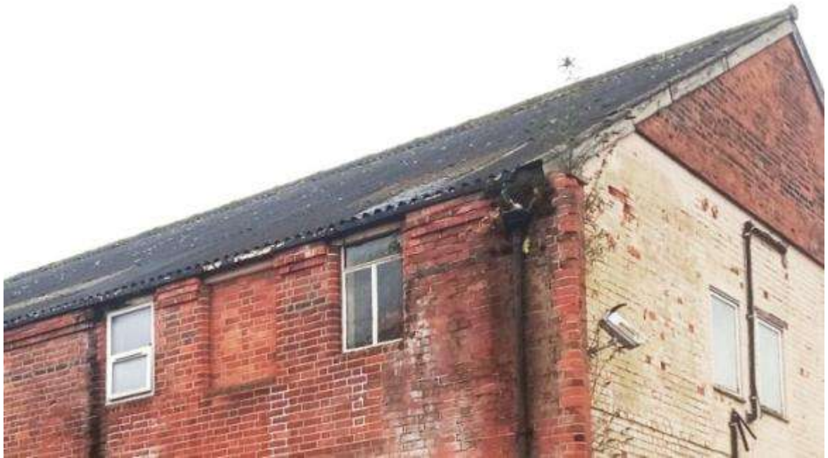
Fig 3.2.6: Eaves to north block (73)
